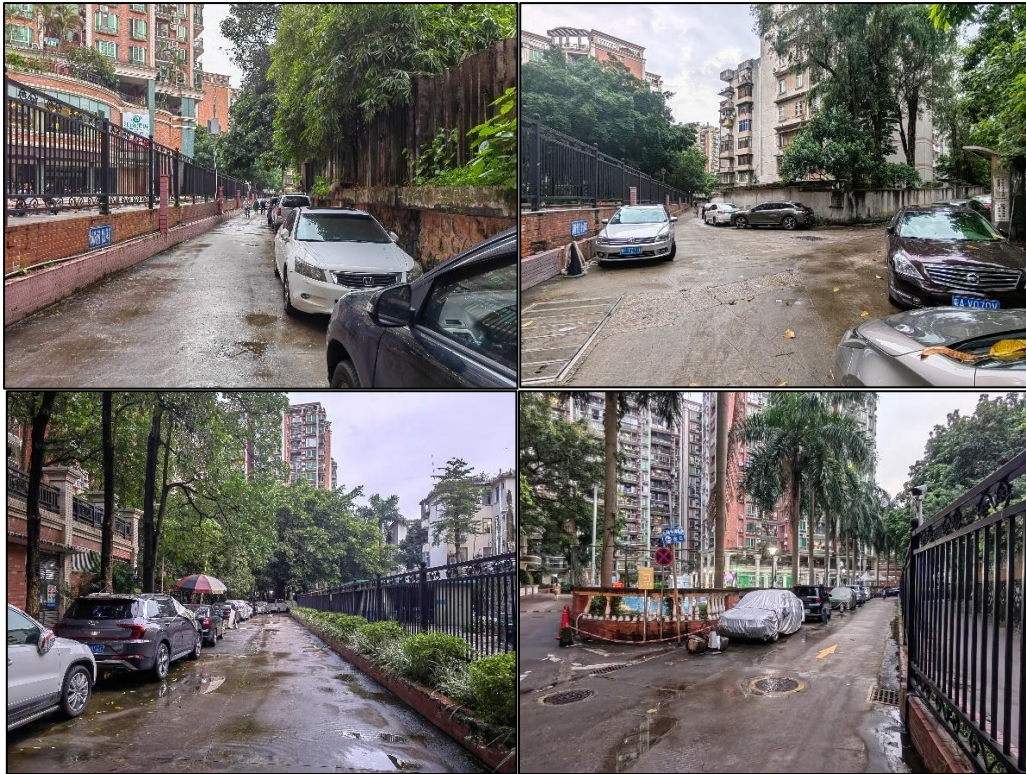
Figure 4-30 Status of roads in the site (Source: Photographed by the author)
