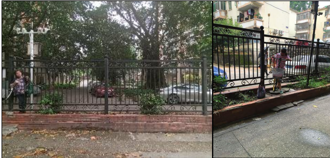
Figure 4-31 Residents sawed through the fence for access
