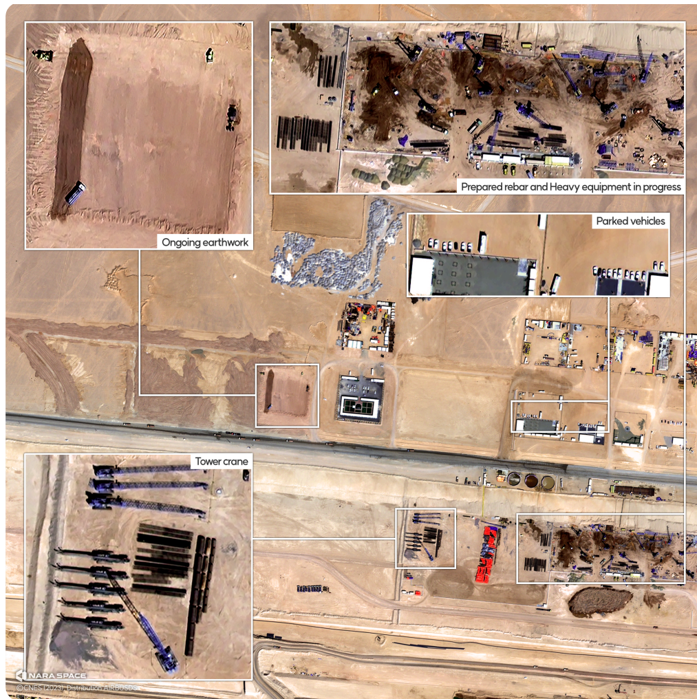
Figure 14. Satellite image of the construction site of the line (source: BBC.com )
