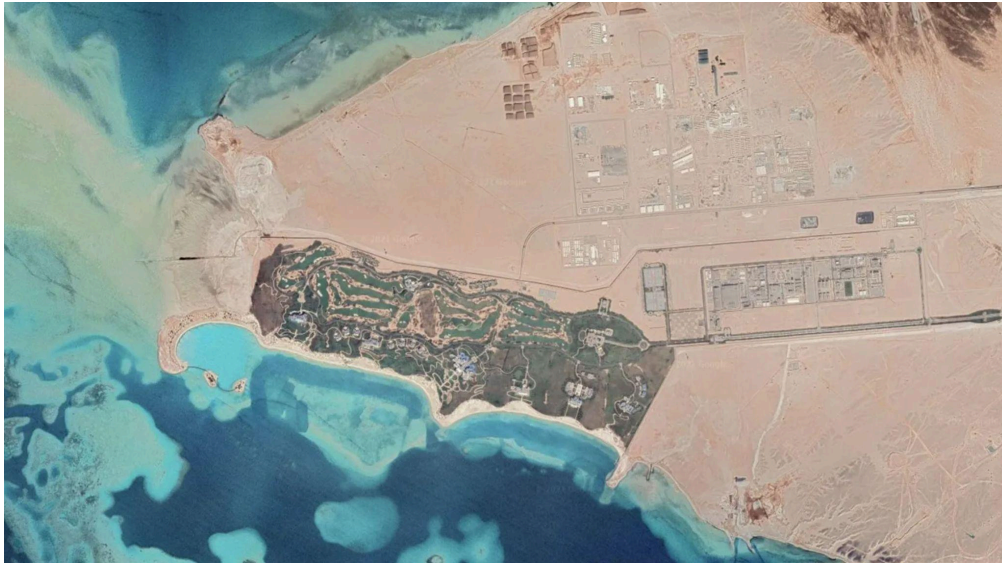
Figure 3. Part of NEOM has been built - including a golf course and a helipad (source: www.bbc.com)
