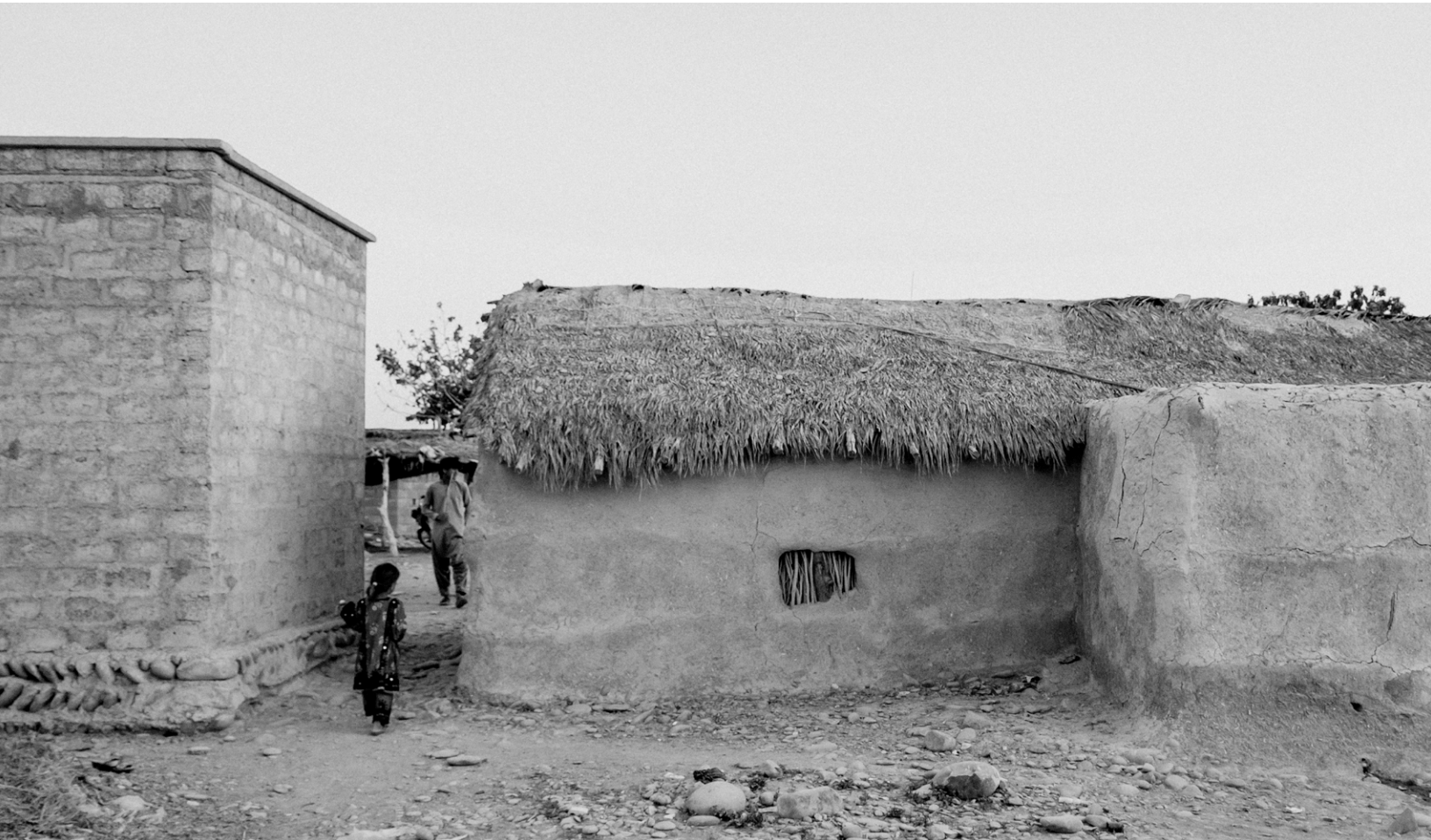
“Two Houses, one built by Khesht and Kapar Roof Structure (right) and another with Concrete Block Walls and Concrete Roof (left). Kahnanikesh” Photo by the Author.
