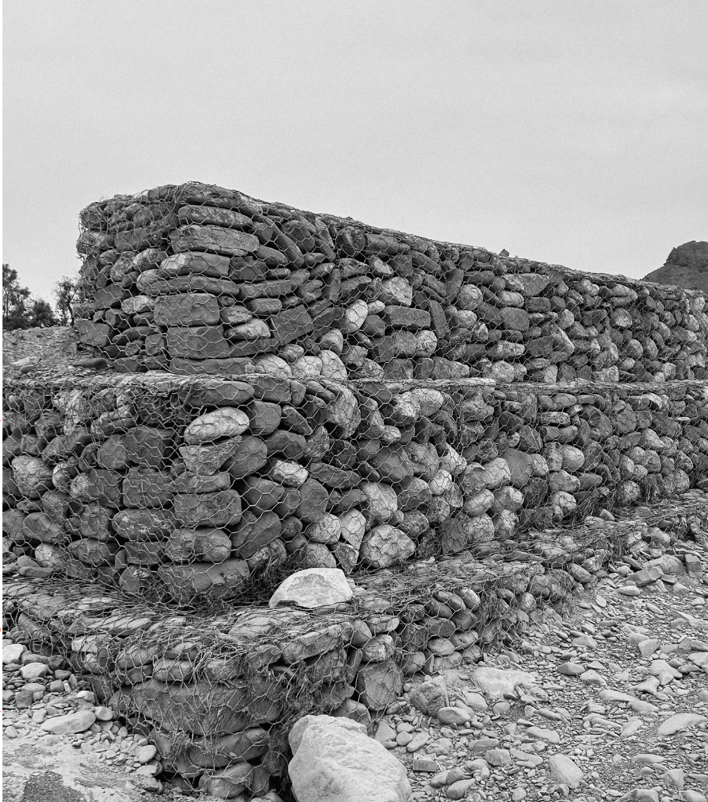
“Flood protection using river boulders. Dooshinkouh” Photo by the Author.
