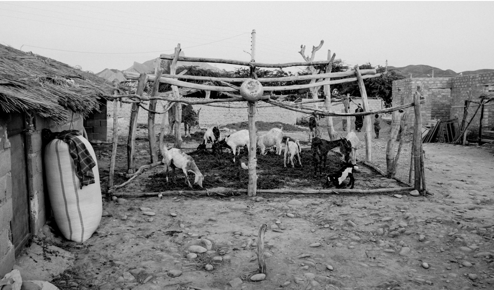
“Outdoor animal shed using tree trunks structure. Kahnankesh” Photo by the Author.
