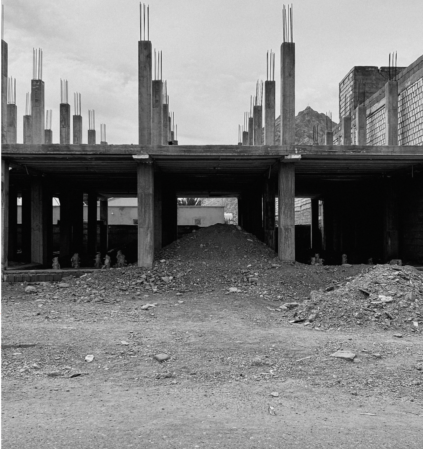
“A building under construction with cast-in-situ reinforced concrete (RC) frame structure. Bent, Nikshahr Country” Photo by the Author.
