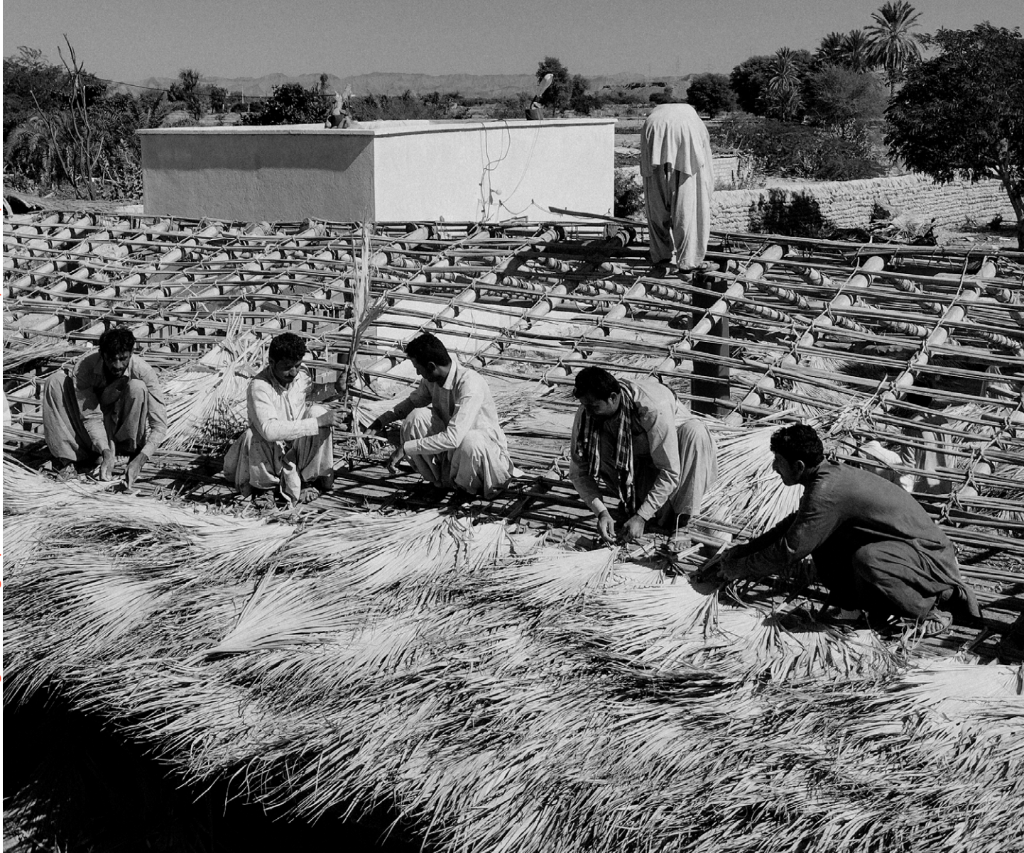
“Constructing a roof using Kapar structure. Kahnaniqesh, Dashtyari Country” Hadi Aledavood. 2023. 1
