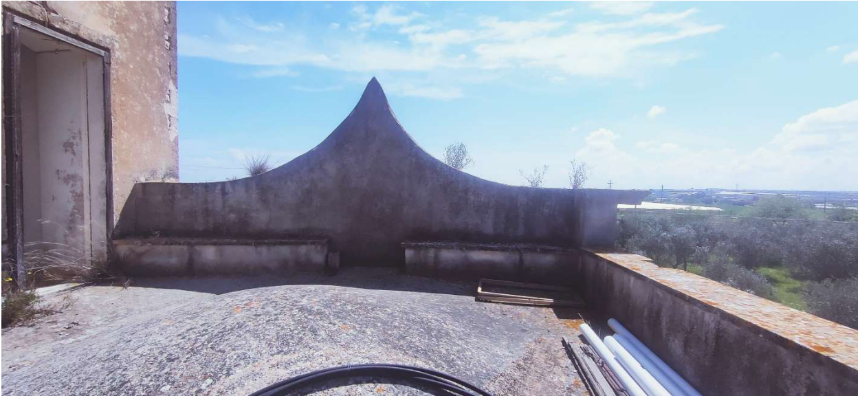
Photo 5-13: View from the terrace of first floor , right above the chapel. The extrusion of the dome is visible in the photo.
