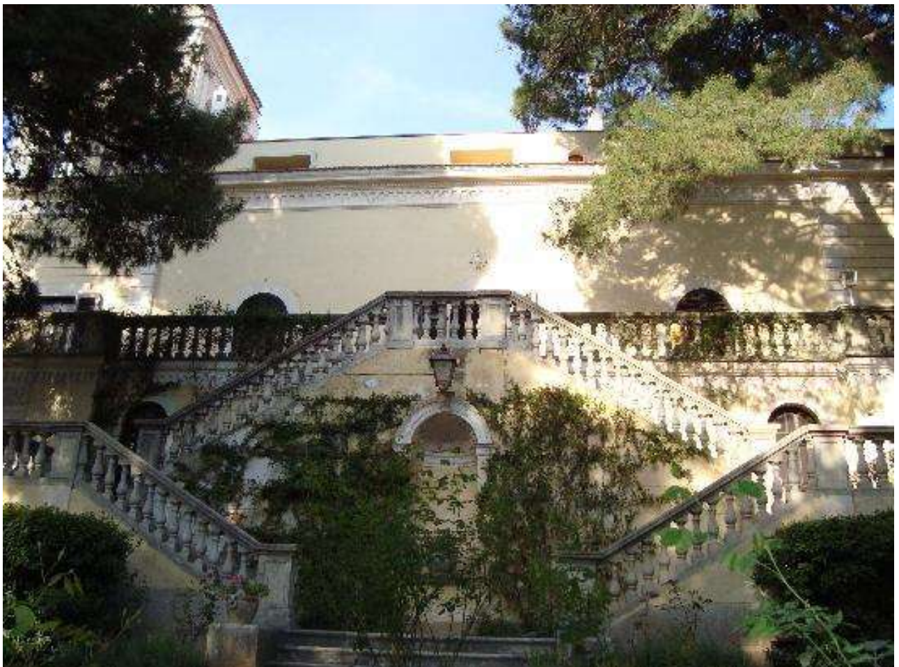
Photo 3-3: COUNTRY HOUSE CEFALICCHIO-CANOSA DI PUGLIA (source: Google)
