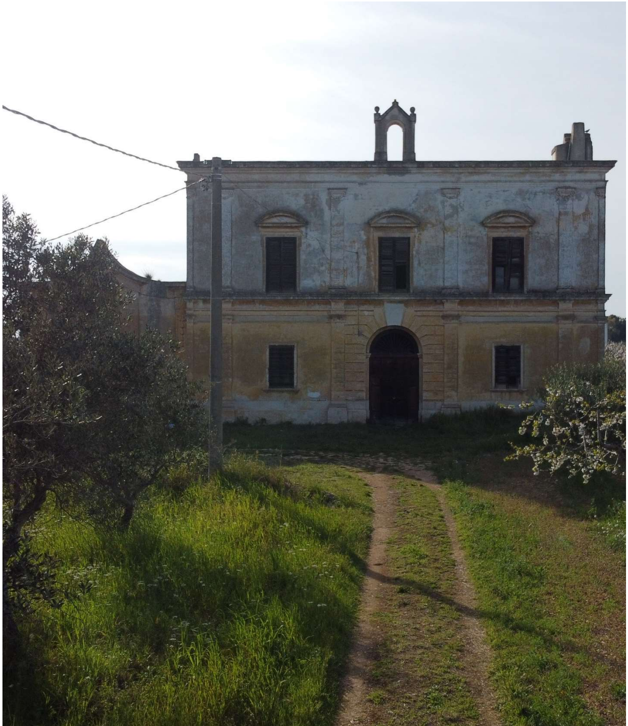
Photo 5-1: Front view of the main elevation of the Masseria Martinelli (Picture courtesy: Domenico Tribuzio)
