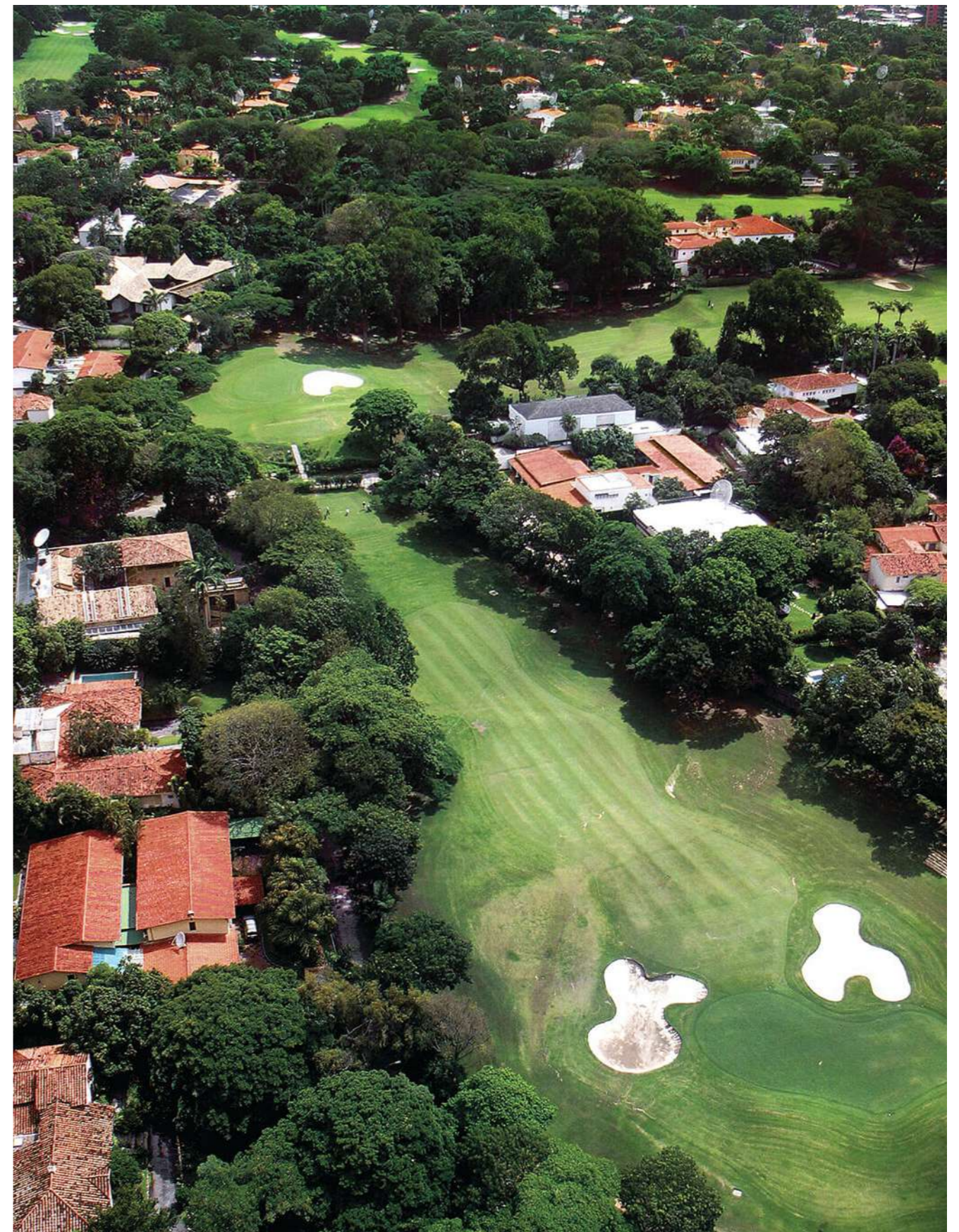
Fig. 125 - The Caracas Country Club Golf Club is a landmark residential development in Caracas, blending urban design with the valley's natural landscape. The project, initiated with the 1929 demolition of the Blandín House, was developed on land that once belonged to the area's first coffee plantation. The Blandín Syndicate, composed of prominent families and advised by Nelson Rockefeller, employed the Olmsted Brothers Associates, famed for New York's Central Park, to design the landscape. They utilized the scenic qualities of the land, preserving large trees and views of the surrounding valley and Ávila peak. The golf course, designed by C. H. Banks and built in two stages, respected the area's topography, incorporating existing tree-lined pathways and preserving century-old trees. This unique development is recognized for its integration of urban and natural elements, with its plans archived at the Frederick Law Olmsted National Historic Site and the Library of Congress in Washington D.C. - (www.guiaccs.com)
