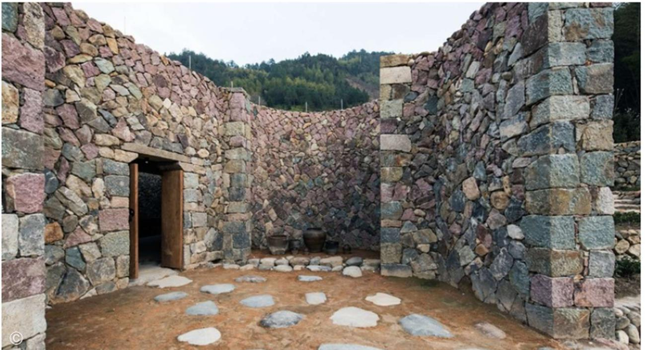
**Figure 3** Stone Masonry Structure (Hakka Indenture Museum)
