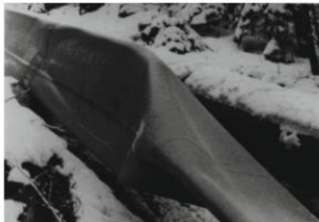
Figure 4 The fallen penstock of Lutschinen Hydroelectric Power Plant
