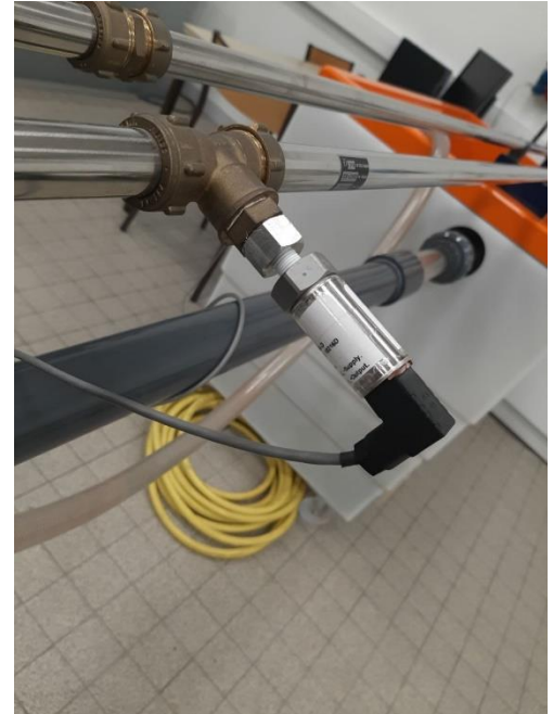
Figure 14 A pressure sensor installed in the middle of the second pipe
