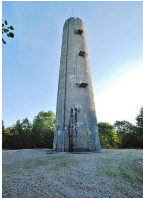
Figure 5 Lastioules equilibrium chimney [7]
