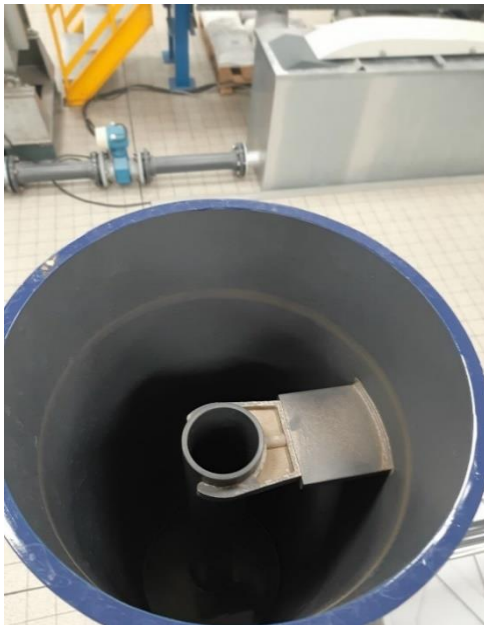
Figure 9 Spillway inside the Water Reservoir
