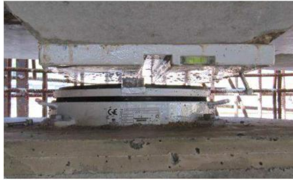
Fig.1.4. Detachment of bearing top's plate
