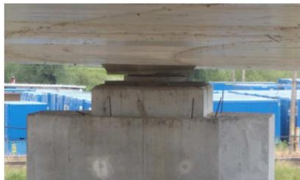
Fig.1.6. The effect of bearing overload
