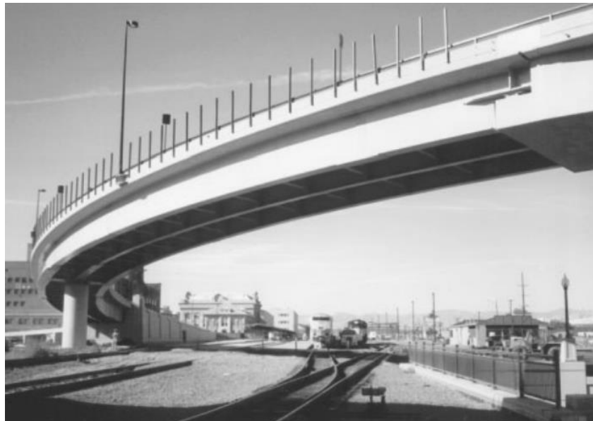
Figure 1.1. Curved I-girder viaduct
