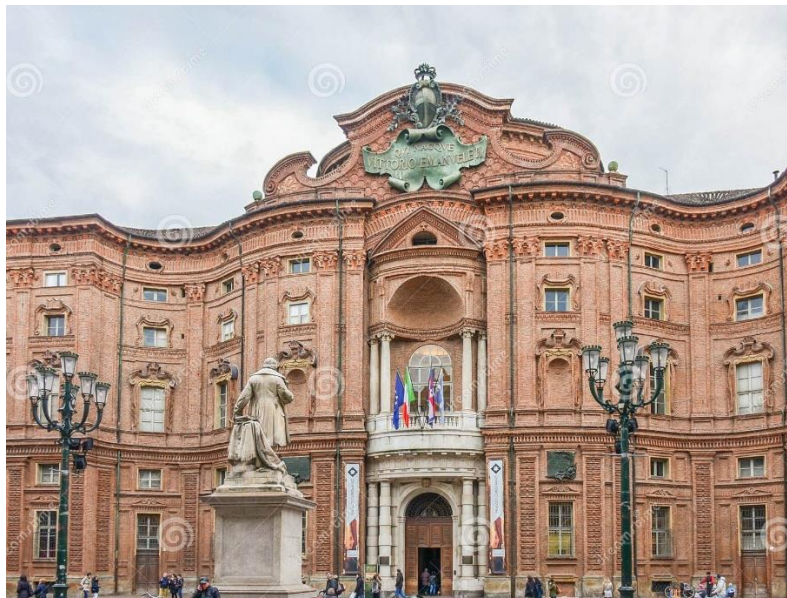
Figure 1.4 Palazzo Carignano of Turin- masonry structure.
