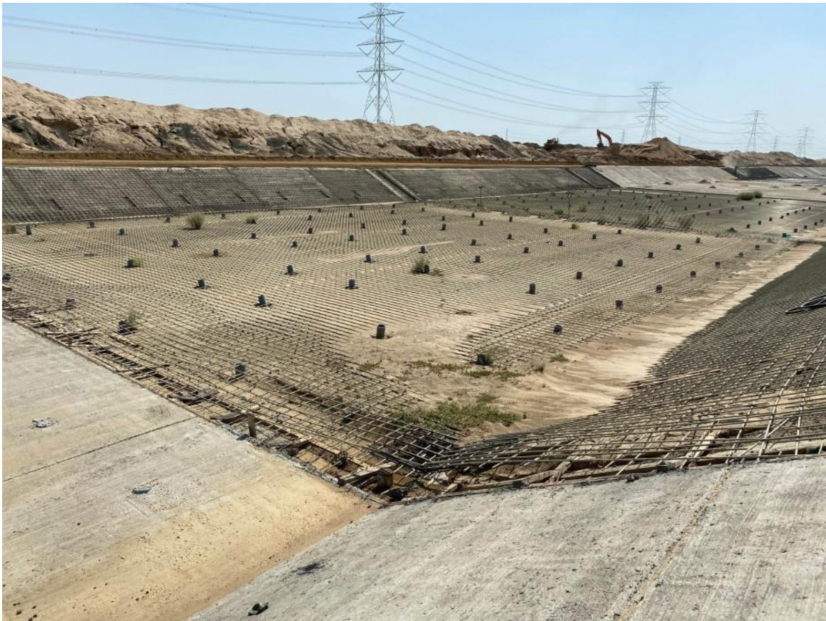
Figure 2.9 Jizan Flood Mitigation Channel GFRP Reinforcement
