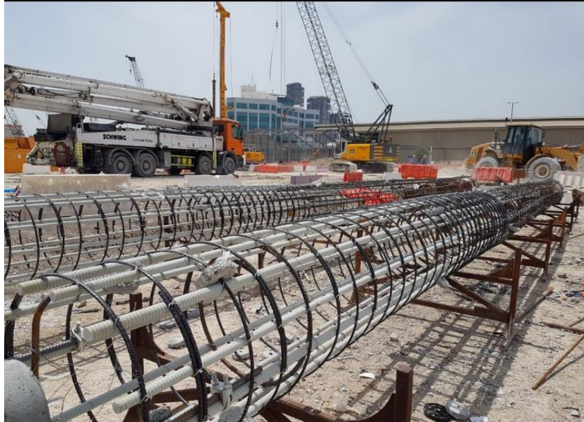
Figure 2.13 GFRP piles reinforcement.
