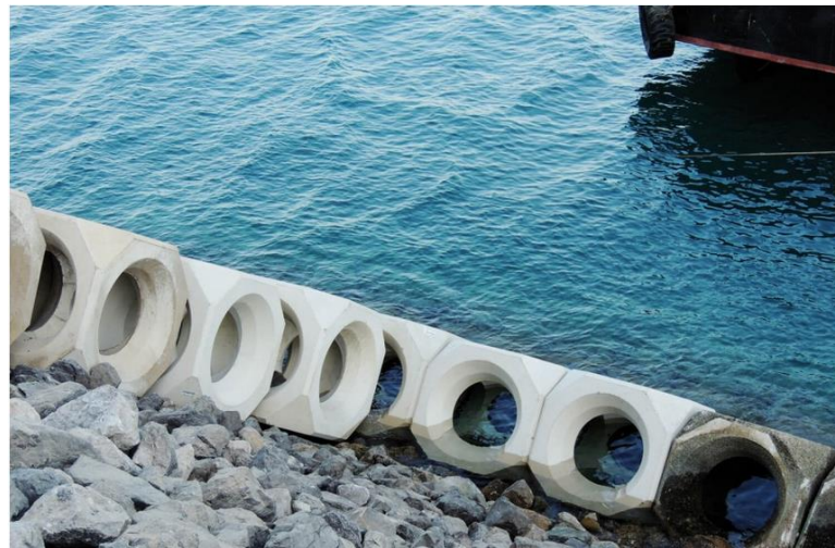
Figure 2.11 SHED concrete armor units
