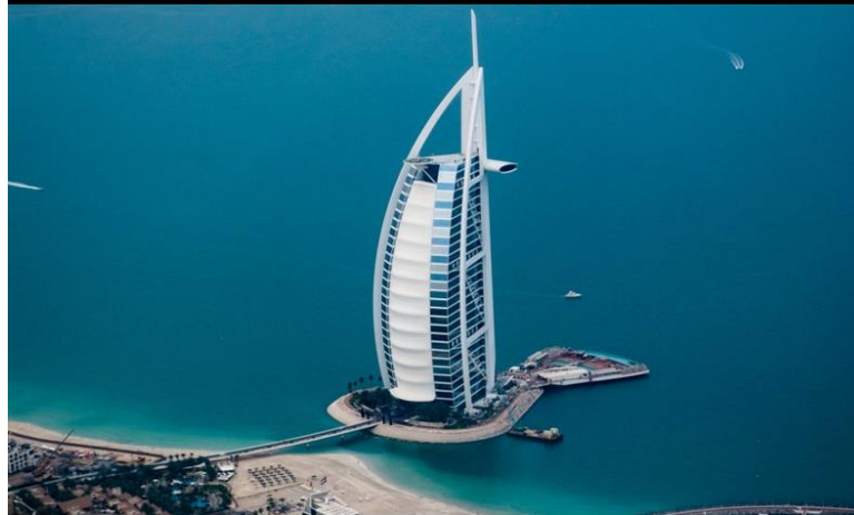
Figure 2.10 Seawall Strengthening the iconic Burj Al Arab:
