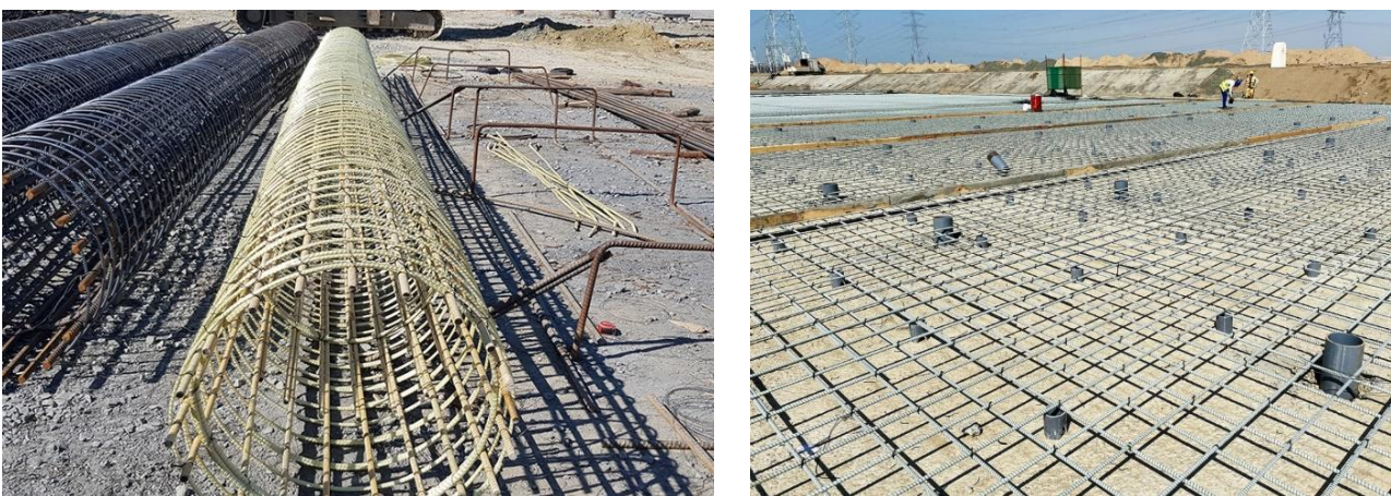
Figure 2.7 Bored pile in GFRP The Jizan Flood Mitigation Channel in GFRP
