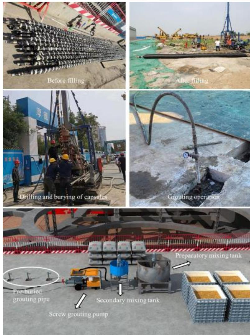
Figure 10: Capsule Grouting Equipment and Procedure (Zheng et al., 2022)
