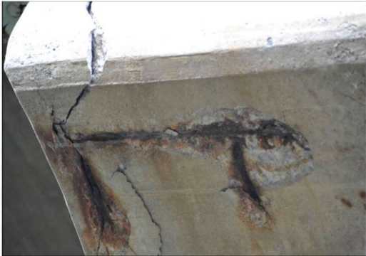
Figure 8-Corrosion (Janamian & Aguiar, 2023)
