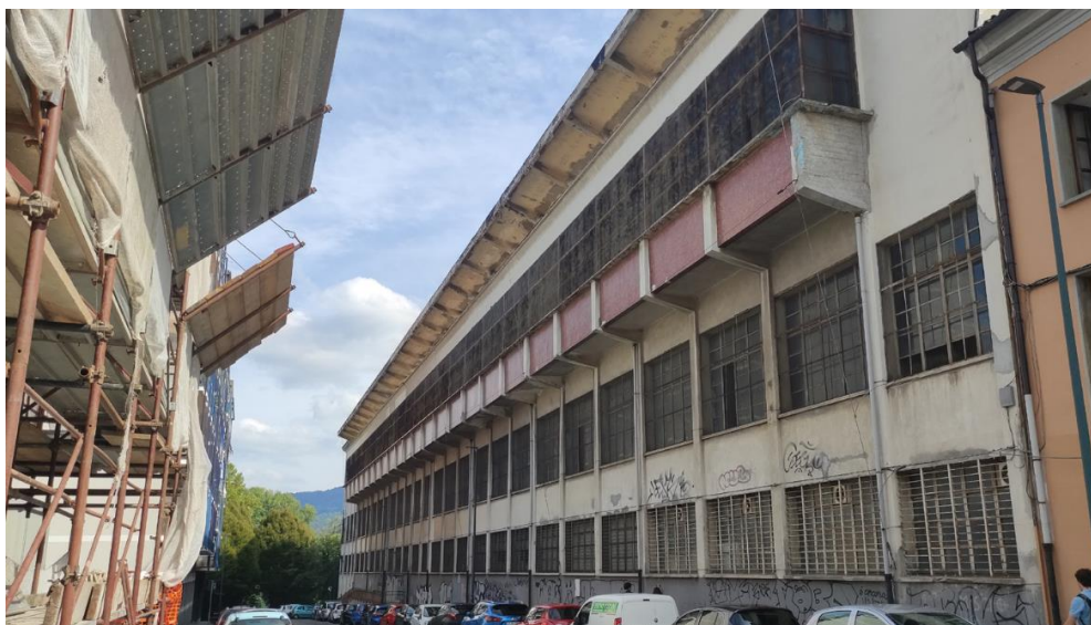
Figure 4.2.5 Building no.8's north façade (Google Earth).
