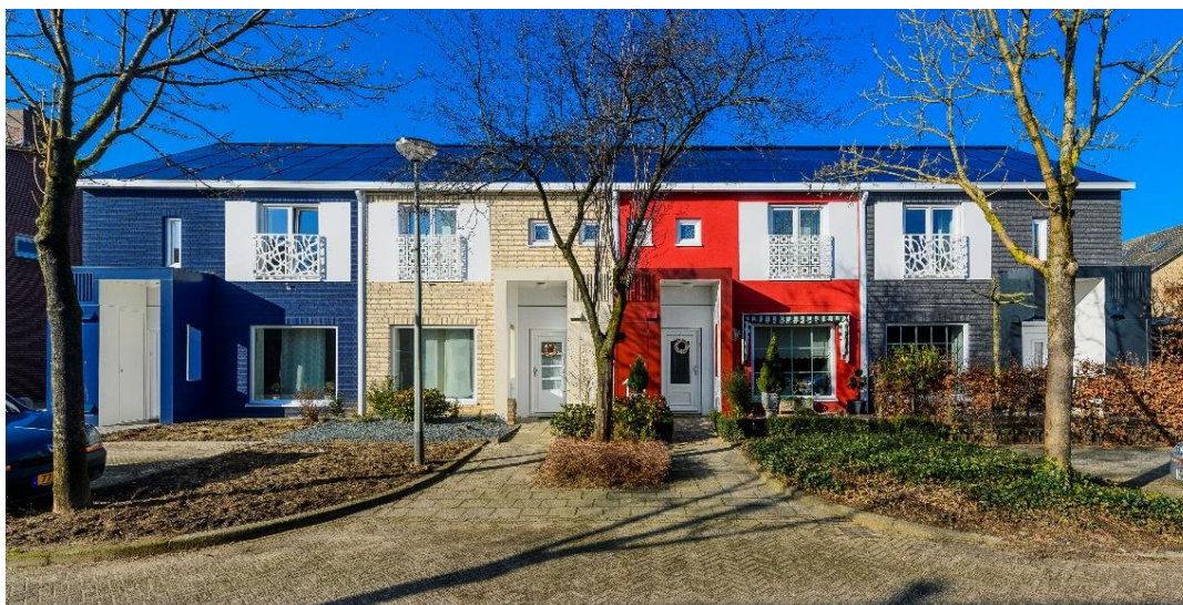
Figure 2.3.2 Parellelweg, Melick after renovation ( https://www.energiesprong.uk/publications ).
