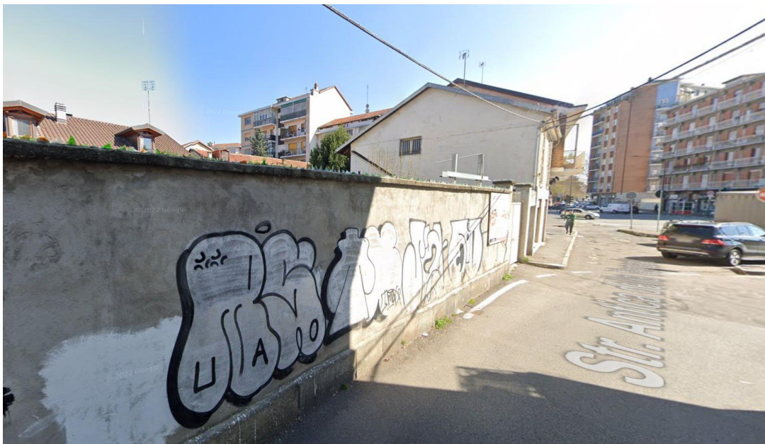
Figure 4.1.3 North façade (Google Earth).
