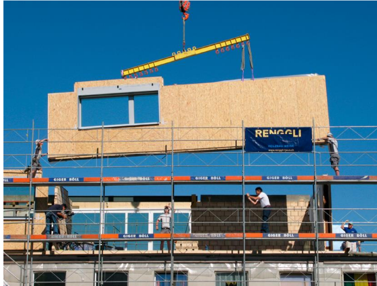
Figure 2.3.1 Mounting a prefabricated, highly insulating façade element.
