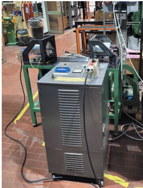
Figure 2.12: Autotransformer that reproduces the grid
