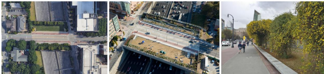
Fig 3-24: Fifth Street Plaza
