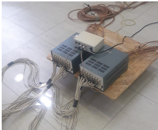
Figure 4.6: Electrets' amplification system with cables
