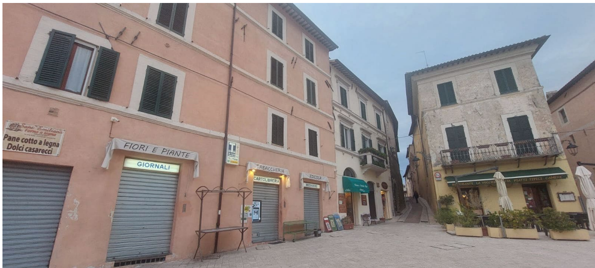
Figure 1: Masonry aggregate building, Treviso, Italy.
