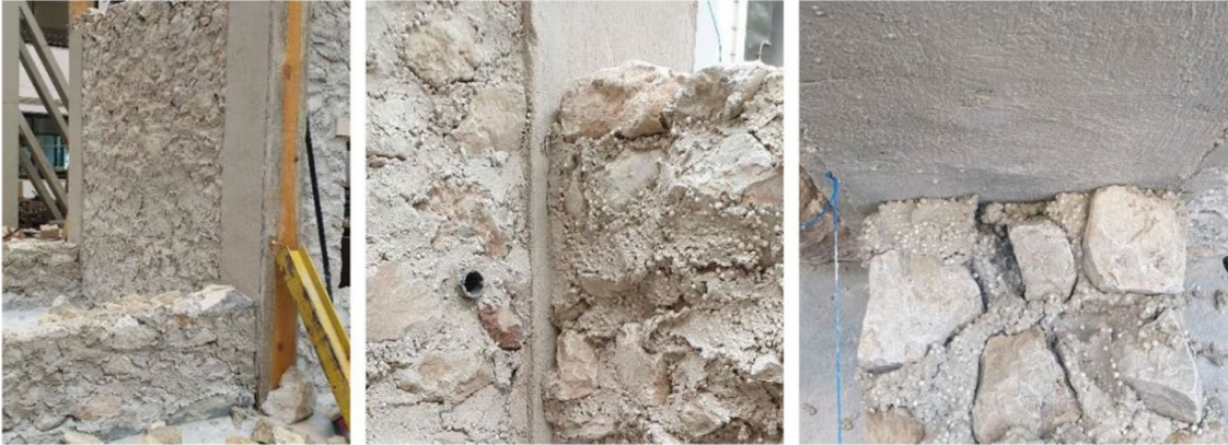
Figure 15: Interface between units in the masonry aggregate (7).
