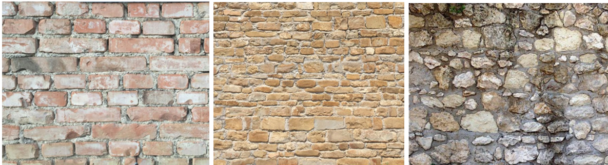
Figure 3: Example of masonry on existing buildings.
