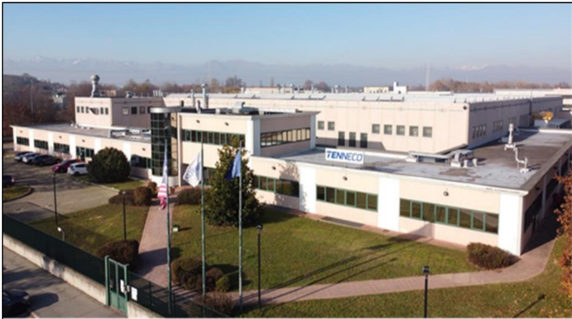
Figure 4, The Tenneco Chivasso Plant
