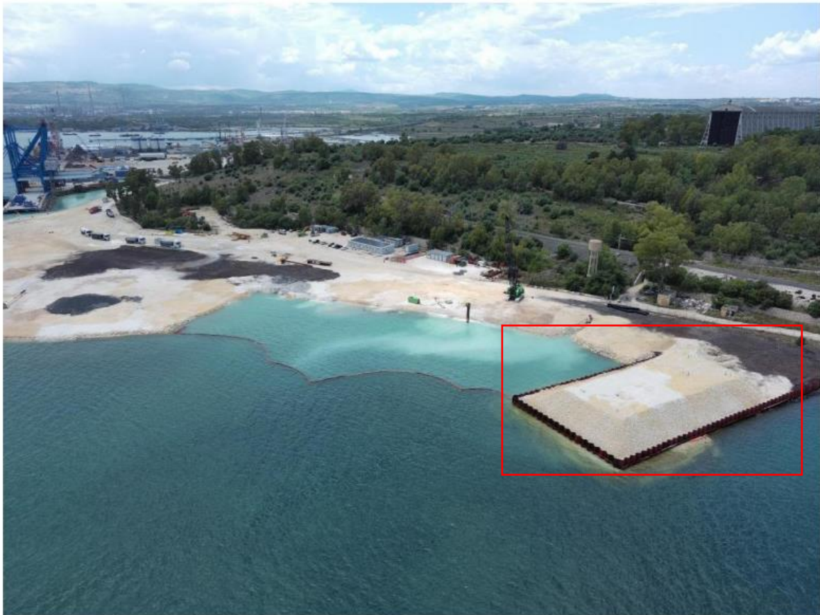
Figure 4.23 Finished test embankment
