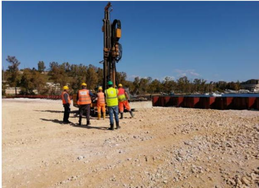
Figure 4.1 Stone column installation on site using bottom feed method
