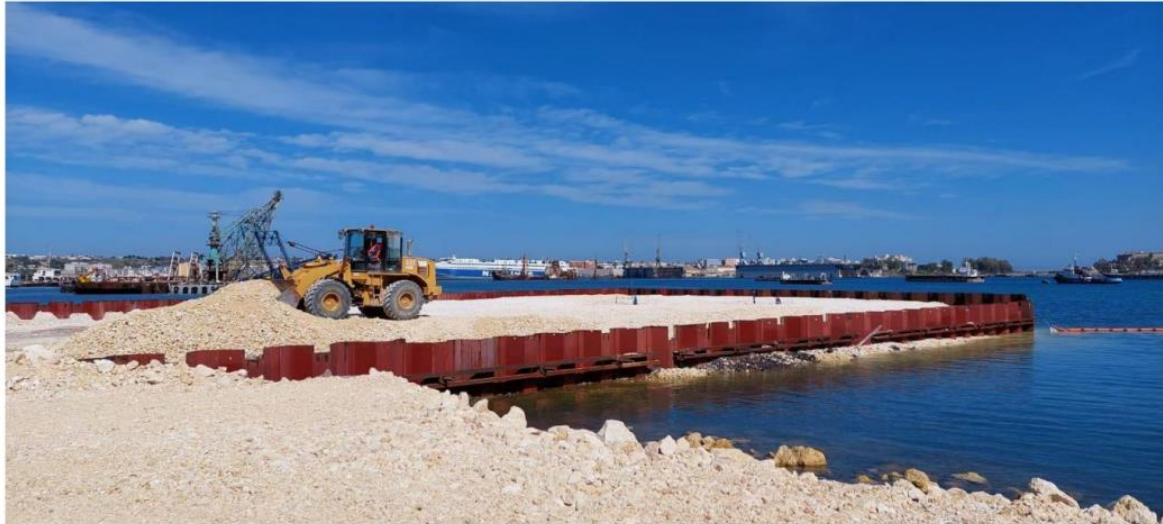
Figure 4.21 First phase filling: finished altitude of +1.00 m above sea level
