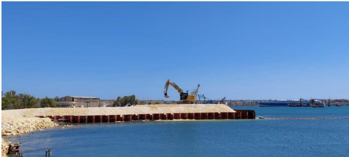
Figure 4.22 Second phase filling: finished altitude +5.20 m above sea level
