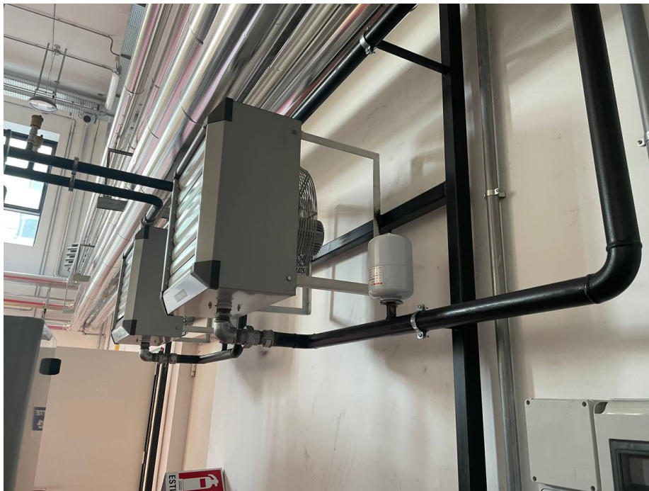
Figure 2-10 Air heaters placement
