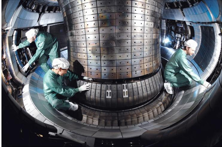
Figure 2.1: Installation work in the plasma vessel. The collector plates of the divertor are seen at the bottom [23].
