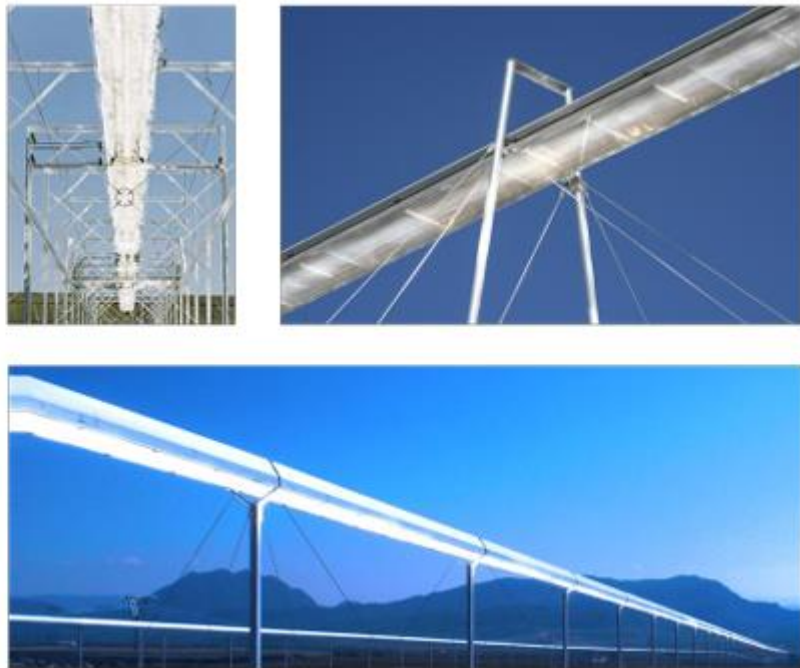
Figure 1.11: Structure of the receiver of the Linear Fresnel Technology [10]
