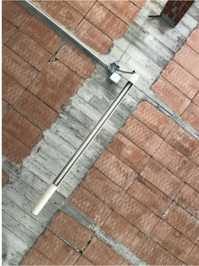
Figure 21. Photo of the floor structure seen from below
