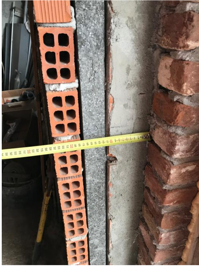
Figure 16. Photo of the wall
