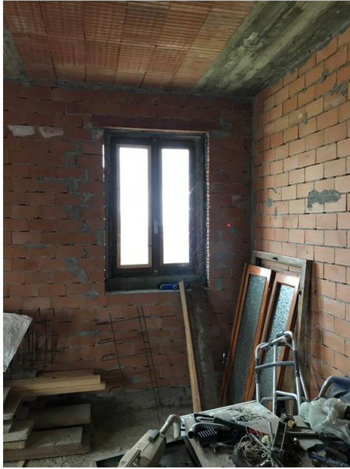
Figure 18. Photo of the Wall
