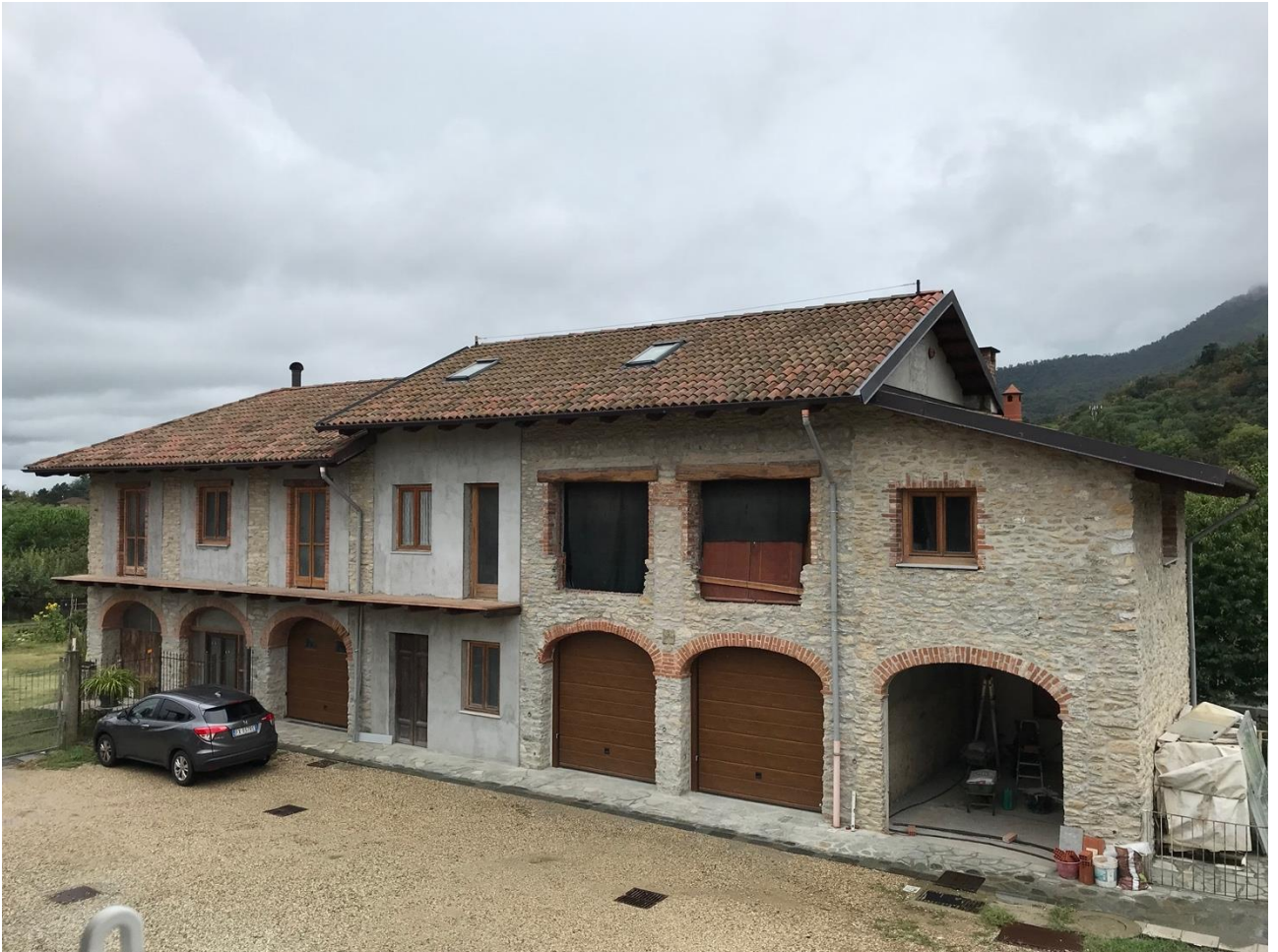
Figure 6. Front view of the building
