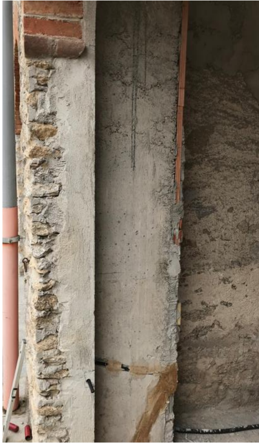
Figure 14. Photo of the wall
