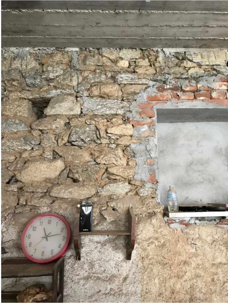
Figure 13. Photo of the wall
