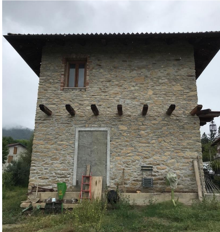
Figure 7. Side view of the building
