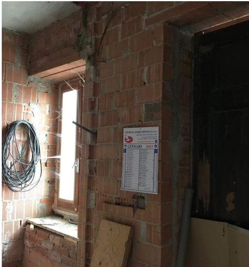
Figure 12. Photo of the wall
