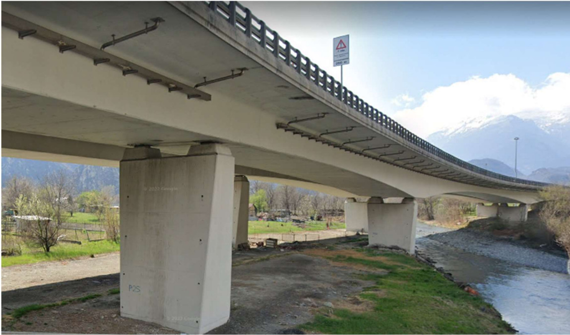
Figure 32 case study Bridge
