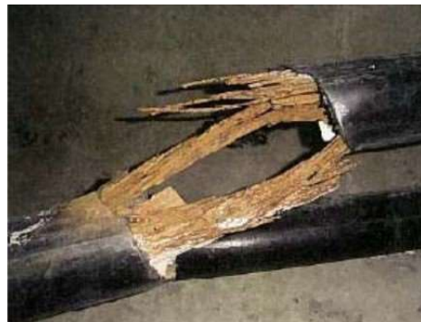
Figure 19 Tendon corrosion
