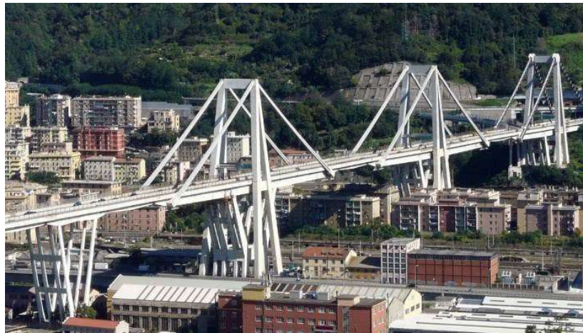
Figure 29 polcevera bridge prior to collapse
