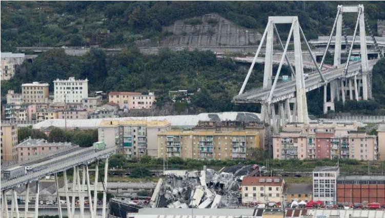
Figure 31 Polcevera bridge after collapse
