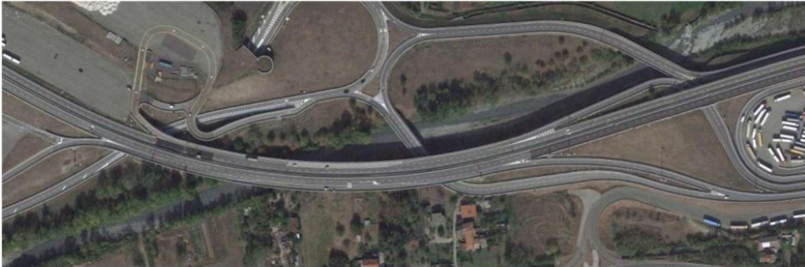
Figure 33 satellite photo of the bridge
