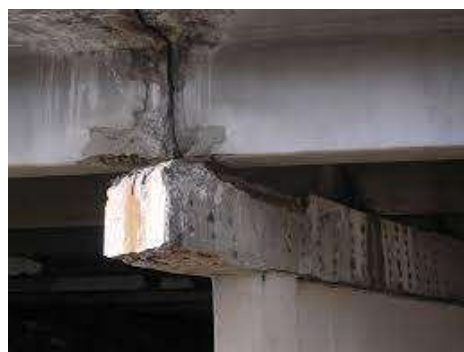
Figure 18 Joint damage
