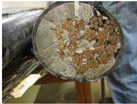
Figure 22 Voids in Ducts
