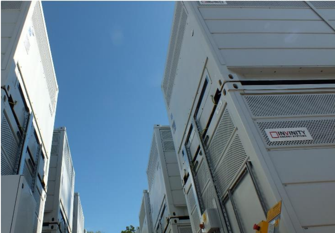
Figure 26: Invinity VFB system Source: invinity.com
