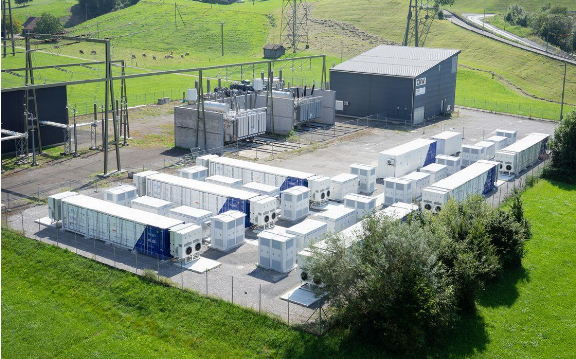
Figure 27: Germany’s largest BESS project to begin construction soon Source: probidenergy.com
