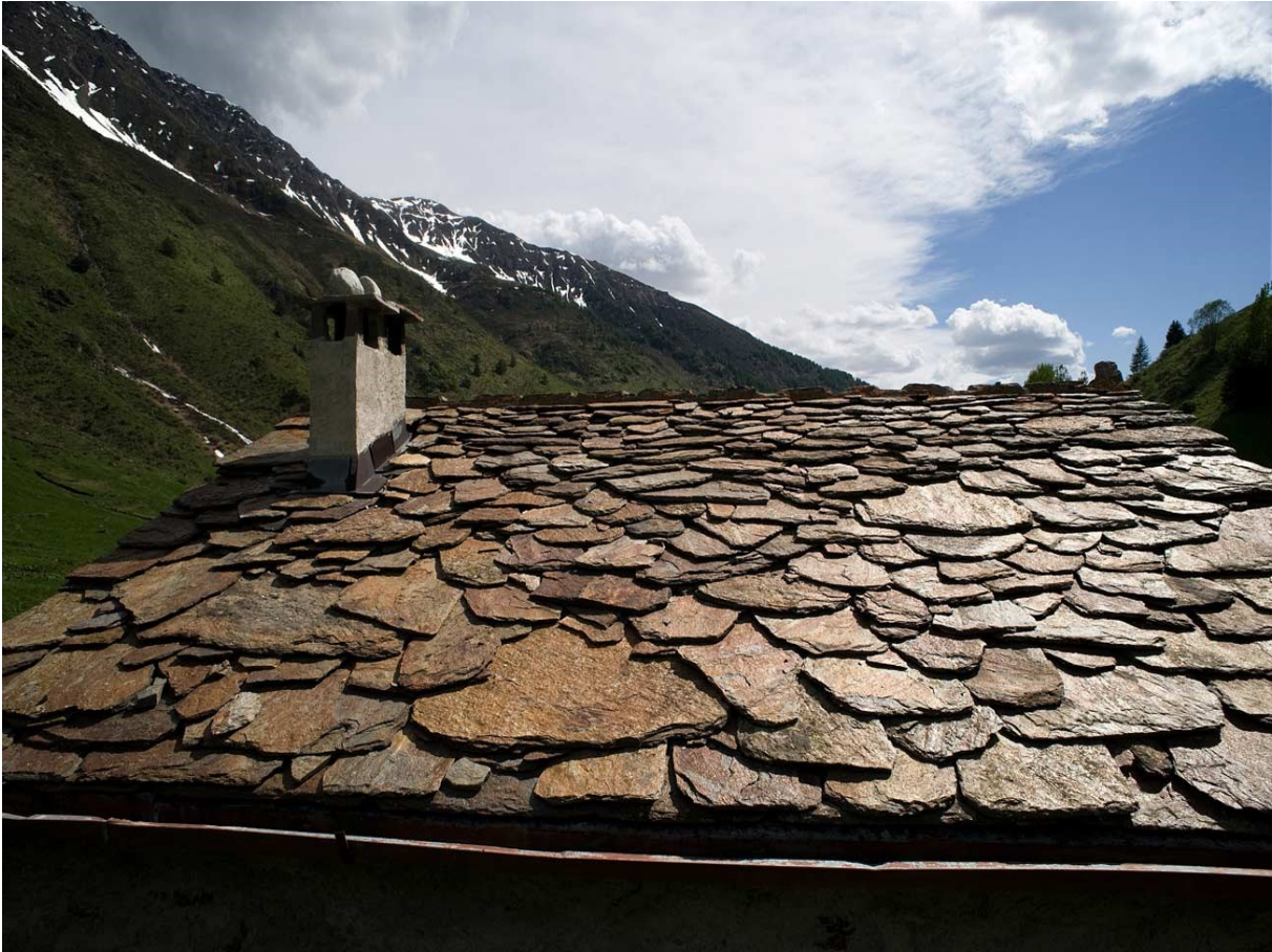
Figure 38 "Lose" stone slabs roof [101]
