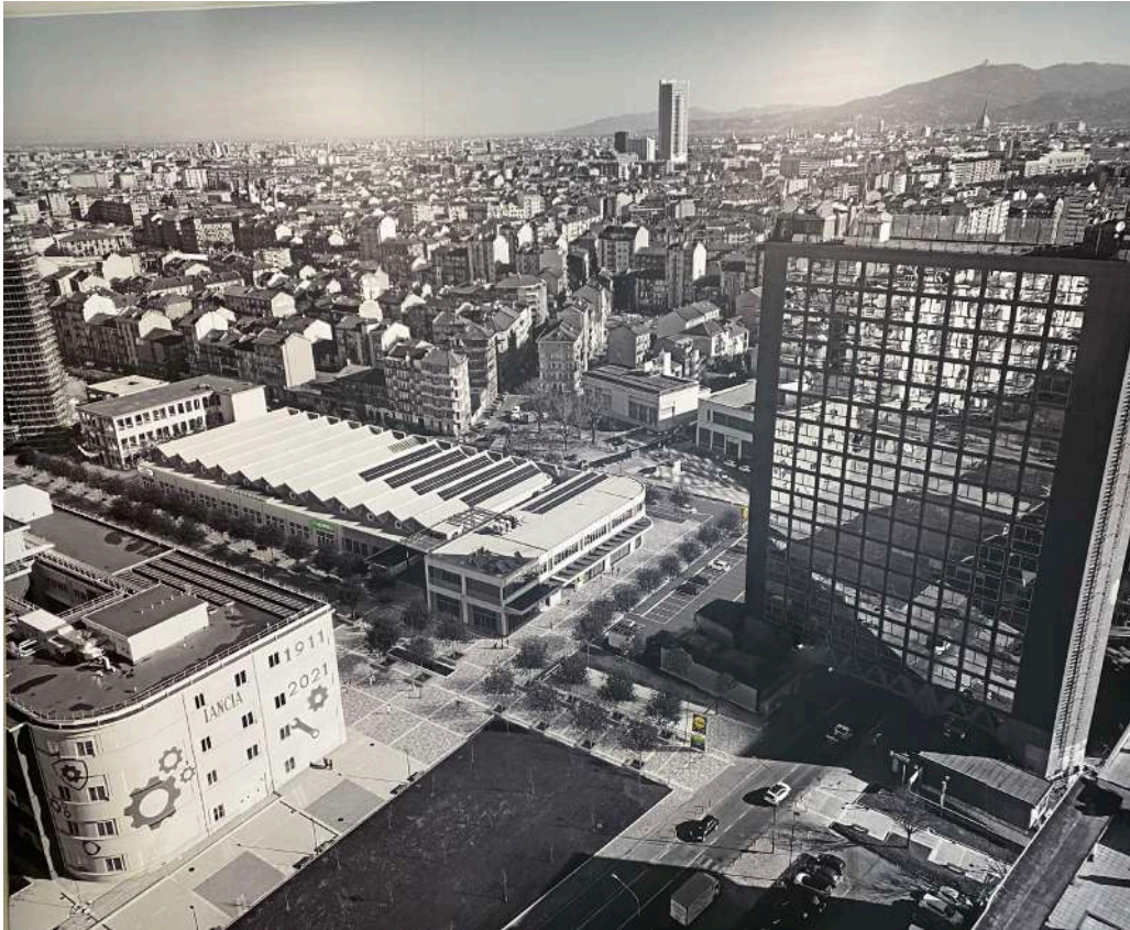
figure21 .current site of lancia Source: Image by the Author in picture located on the Lancia district underground parking
