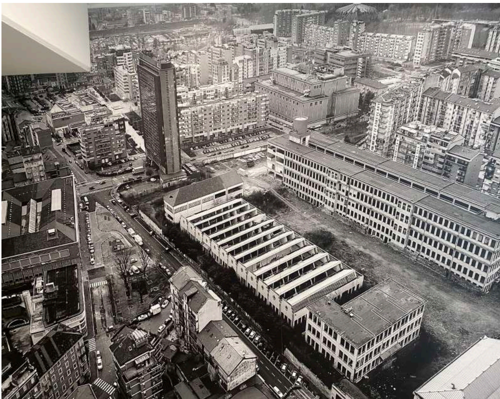
figure 20:Former site of lancia Source: Image by the Author in picture located on the Lancia district underground parking
