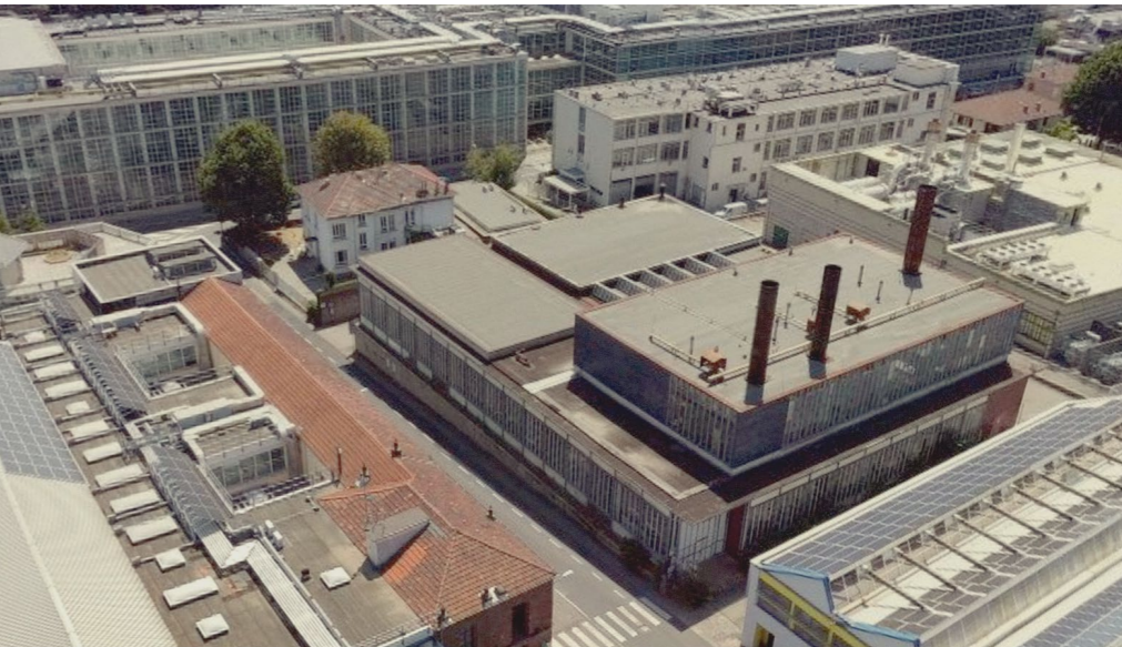
Top View of Centrale Termica
