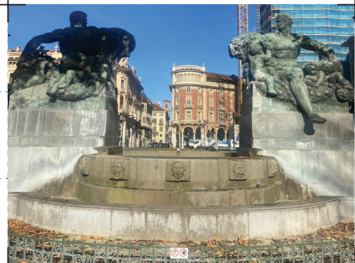
1. Fountain is not well maintained
