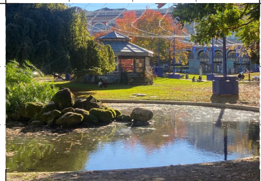
3. The existing water feature is not well-maintained
