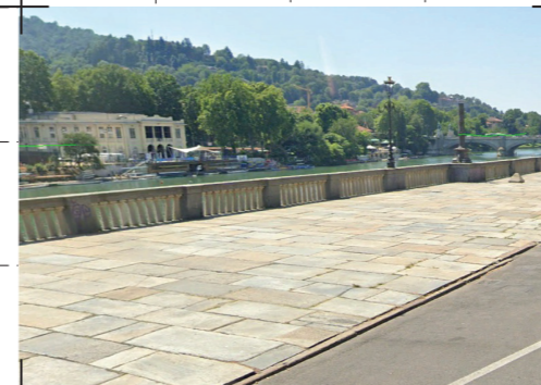
8. Higher than flood level
