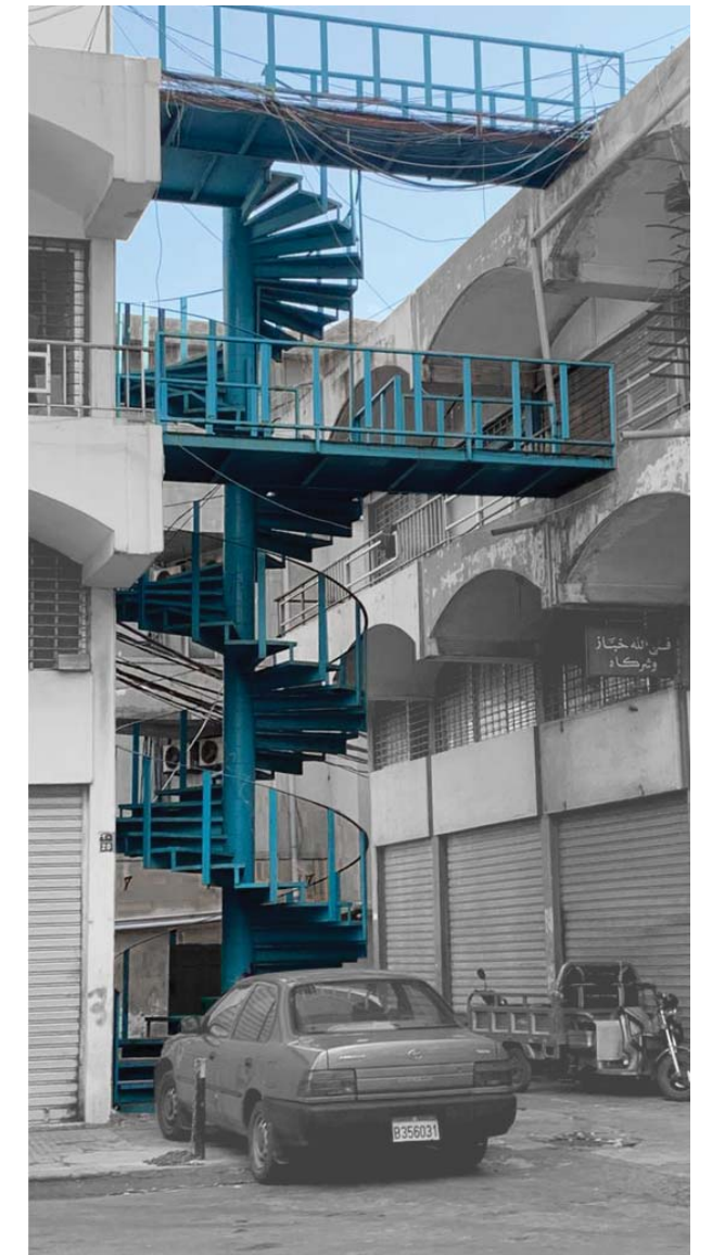
Exterior stair for commercial/industrial building
