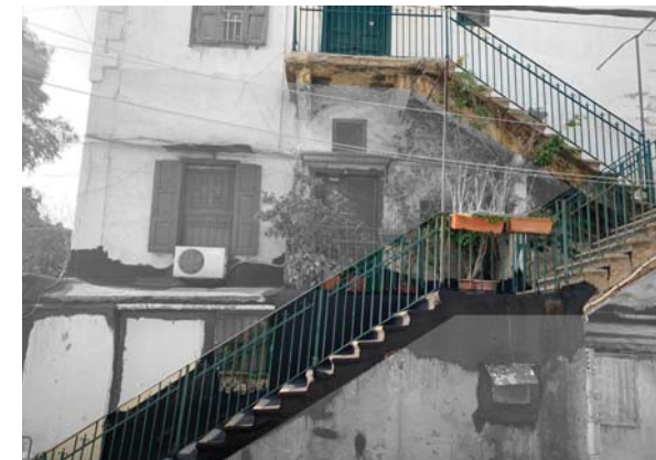
Exterior stair for residential building
