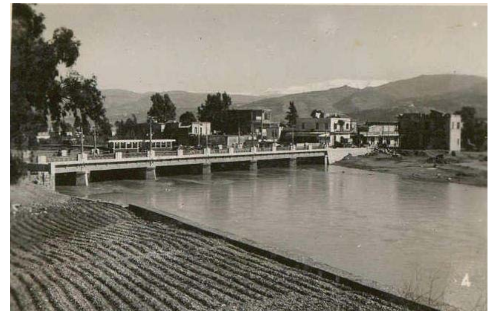
fig.75 Beirut river bridge, Bourj Hammoud, circa 1940's. courtesy of Garo Derounian
