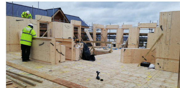
Fig.141. Costruzione del piano primo. Fonte: https://www.self-build.co.uk/blog-timber-frame-erection-facit-homes/
