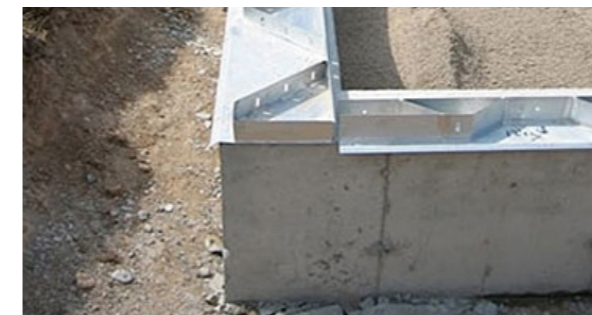
Fig.162. Fondazioni “Portable”. Fonte immagine: https://www.torosteelbuildings.com/options-and-finishes/steel-arch-buildings/foundation/
