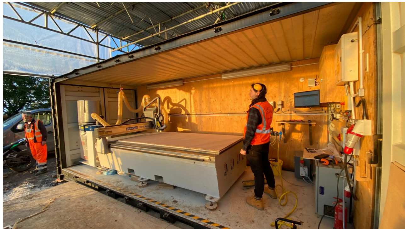
Fig.76. Sistemi produttivo mobile MPF (Mobile Production Facility). Fonte: https://www.facit-homes.com/post/starting-on-site
