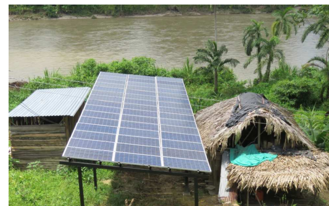
Figure 58. PV Panels installation Source: Colciencias, 2015.
