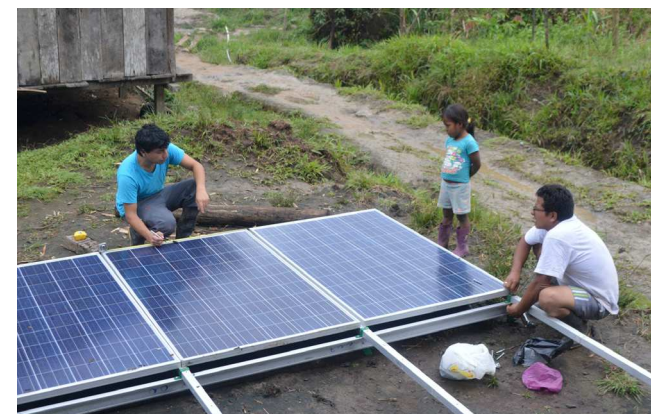
Figure 56. PV Panels installation Source: Colciencias, 2015.
