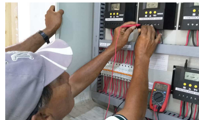
Figure 57. PV Panels installation Source: Colciencias, 2015.
