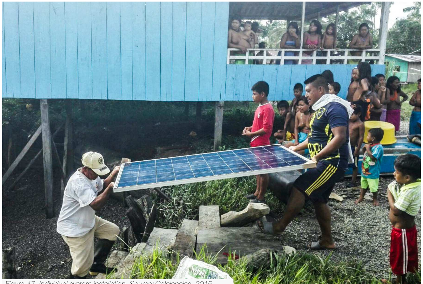
Figure 47. Individual system installation. Source: Colciencias, 2015.
