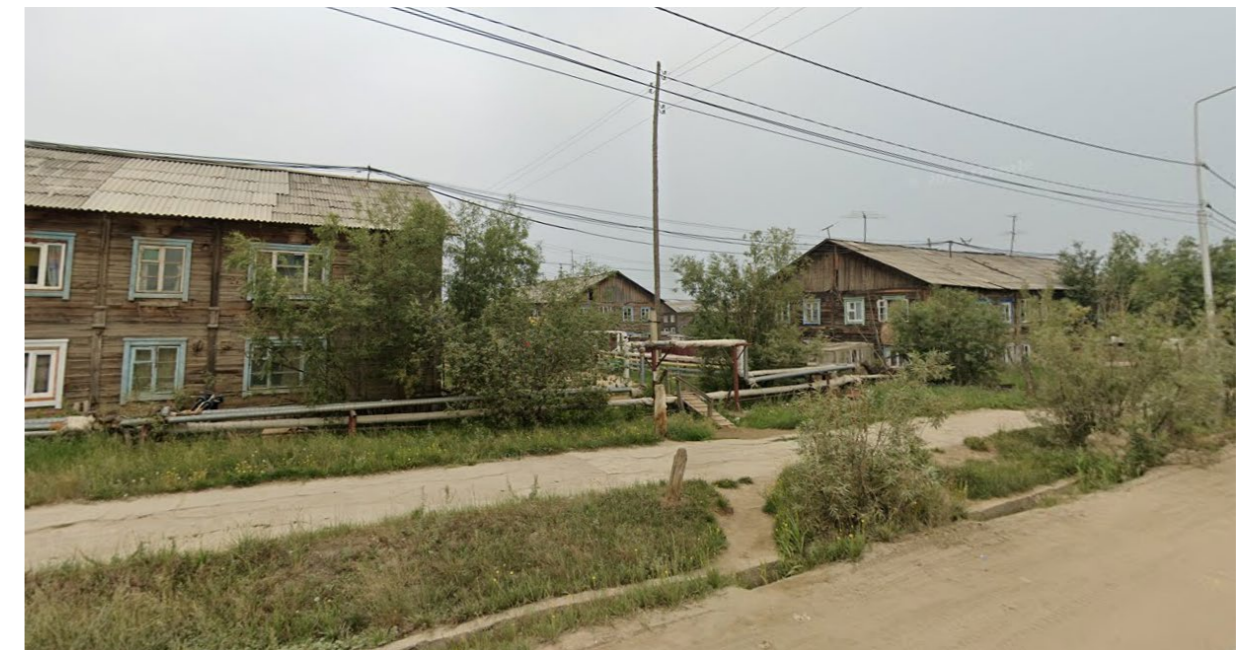
Figure 81: The view from the Google Maps street view shows the condition of the main streets of the area. Despite the devastated condition of the houses, the area is reach with vegetation. Here we can see how existing engineering communications that are located above the ground for permafrost protection, create arches to let locals pass through them. Even though these streets are covered with asphalt we could see the accumulation of dust and sand on them.
