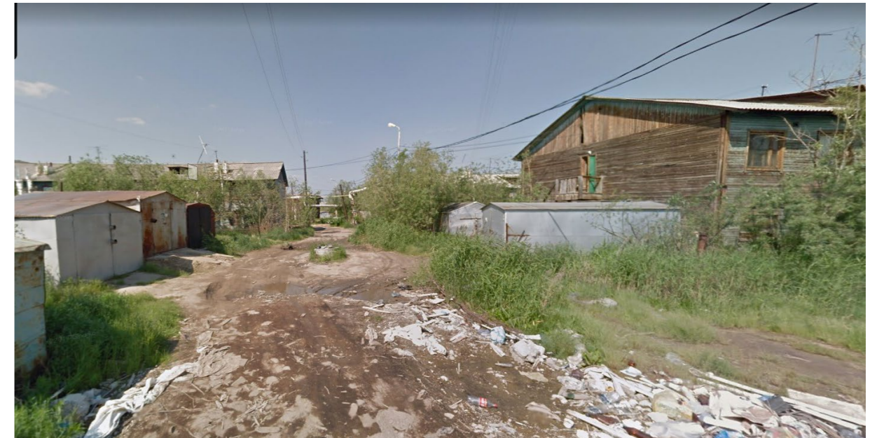
Figure 80: The view from the Google Maps street view shows the condition of the streets of the area. As we can see, some of the streets that lead to the heart of the district do not have any pavement. Rainwater goes down to the ground and provokes permafrost degradation. Uneven ground, pits, and paddles are the signs of permafrost degradation. Moreover, as we can see poor management of the district creates heaps of garbage around the areas. The area is built predominantly with two floors of wooden buildings (we can see them on the right part of the photo and its background). On the sides of the road, we can see garages that are used by locals not only for the cars but also for the storage of the goods.
