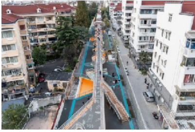
Fig.8: Caoyang Centennial Park, Shanghai, 2022
