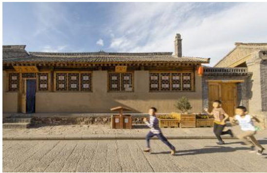
(Fig. 12 The main street after renovation
