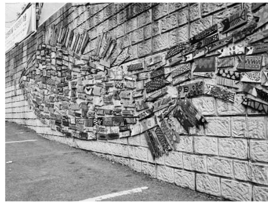
(Fig.18 Renovation of building facades Source: Internet)
