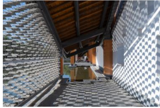
(Fig.24 Internal view of the Corridor Source: https://www.goood.cn )
