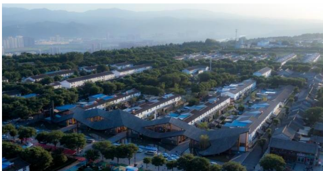
(Fig.1 Overall aerial view of the project after renovation.
