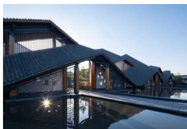
(Fig.19 New Landmark at entrance Source: https://www.gooood.cn )
