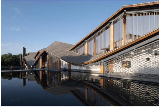
(Fig. 23 External view of the Corridor Source: https://www.goood.cn )
