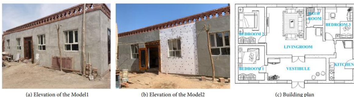
Figure 28 Reference building overview
