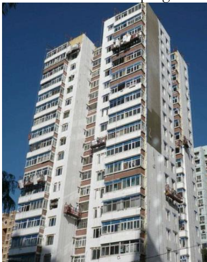
Figure 23 The retrofit picture of Building
