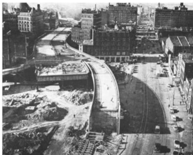
Figure 2. Construction of urban highways in Boston, through the existing urban fabric (Socco, 2009)
