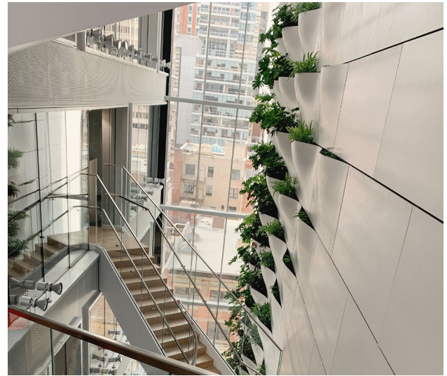
Figure 3.10: Green Wall in Telus Sky Tower from staircase view
