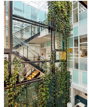
Figure 2.9: Stonnington City Council Office landing featuring a trellis green wall under natural light.
