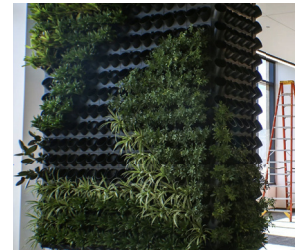
Figure 2.5: Incompleted Pod system living wall for Fasken Oil and Ranch by Green Oasis
