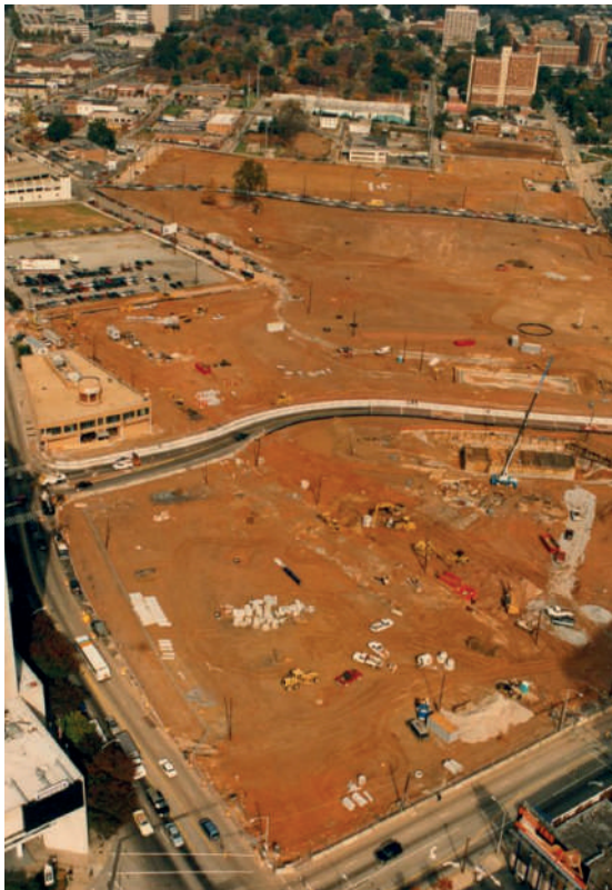
Fig. 31 Centennial Olympic Park construction, aerial view, 1995 46
