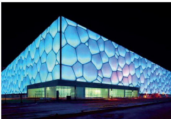
Fig. 70 'Water Cube' National Swimming Center 101
