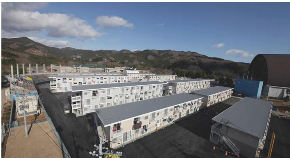
Figure 19: Container Temporary Housing [93]
