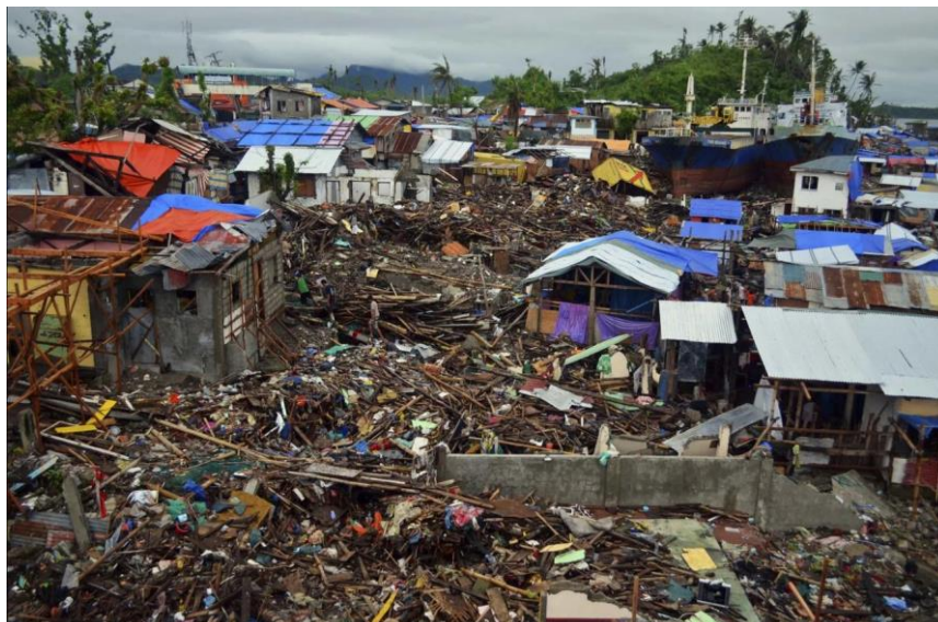
Figure 10: Post Disaster Destruction, Philippines [86]
