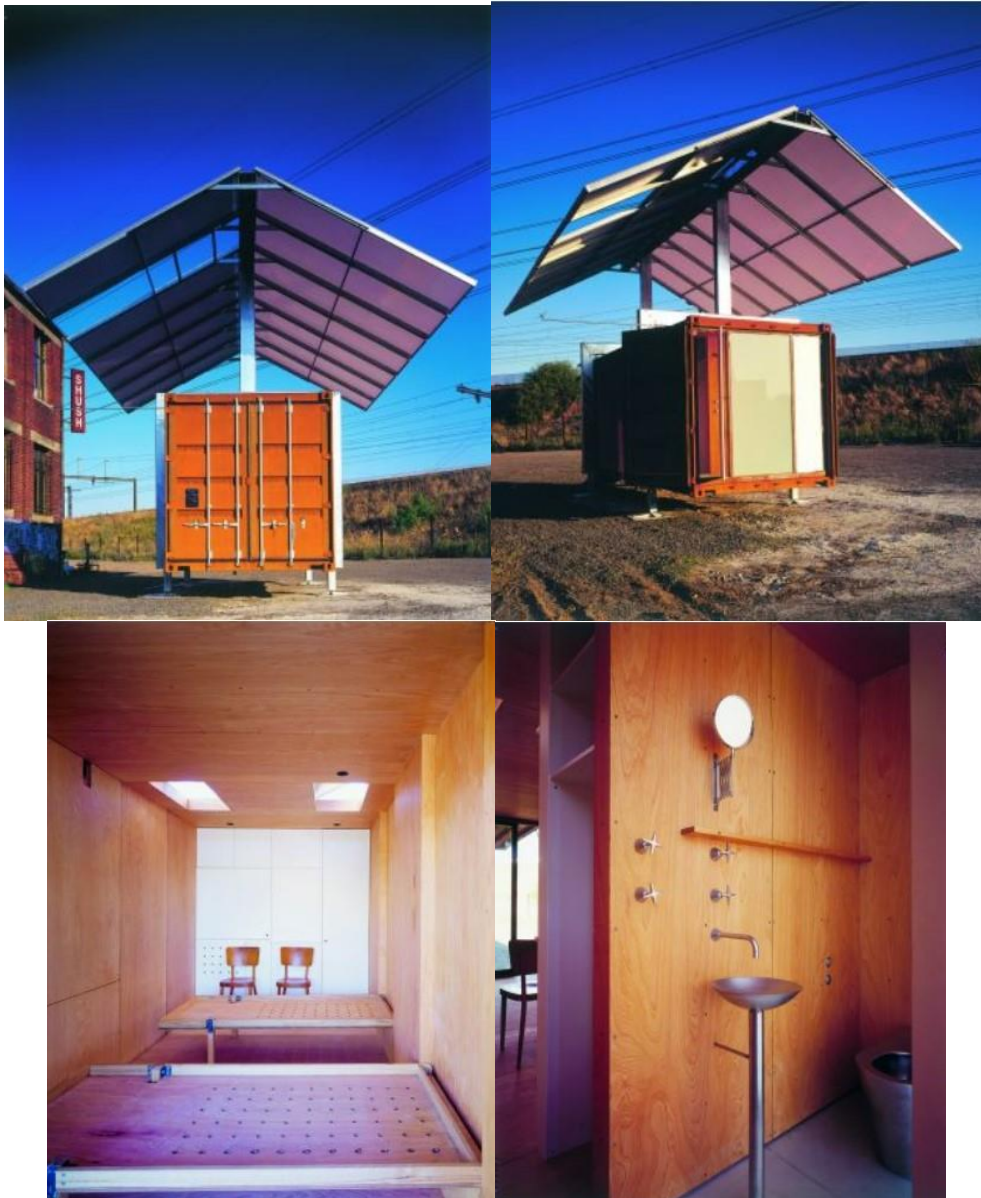
Figure 21: Exterior & Interior, Future Shack [94]
