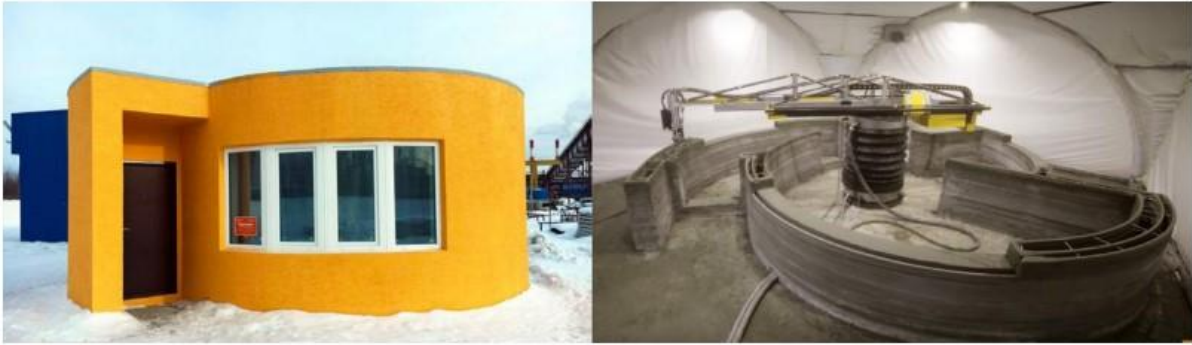
Figure 22: Apri Cor House [95]
