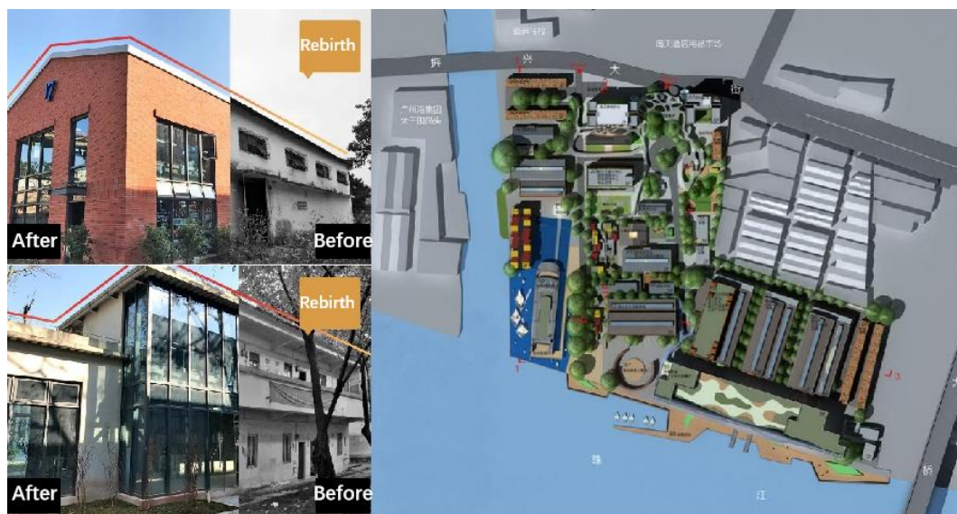
Fig. 3- 13 Before and After Renovation Comparison and Overall Plan Source: https://mp.weixin.qq.com/s/rAqD1VMbxPupYt0Wjb_idA
