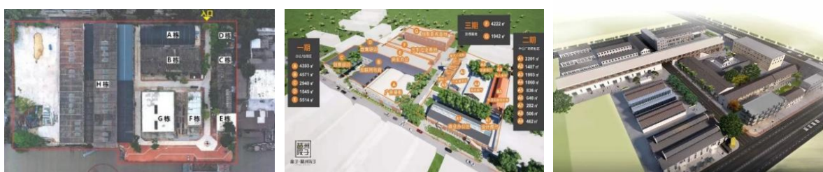
Fig. 3-11 Guangzhou Yulun Factory After Renovation Source: WeChat official account
