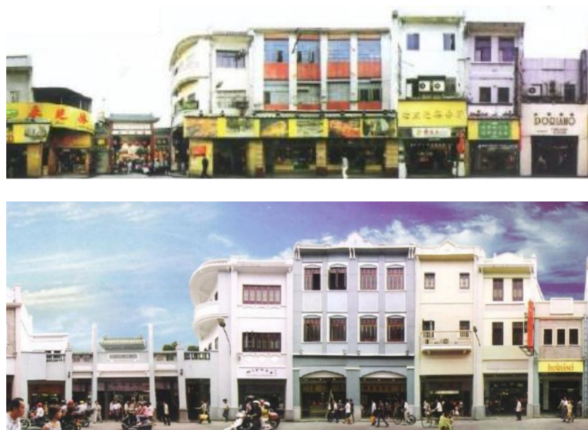
Figure 5-8 Before (top) and After (bottom) the 1998 Renovation Project (Source: Guangzhou Design Institute of Sizhe, Ltd.)
