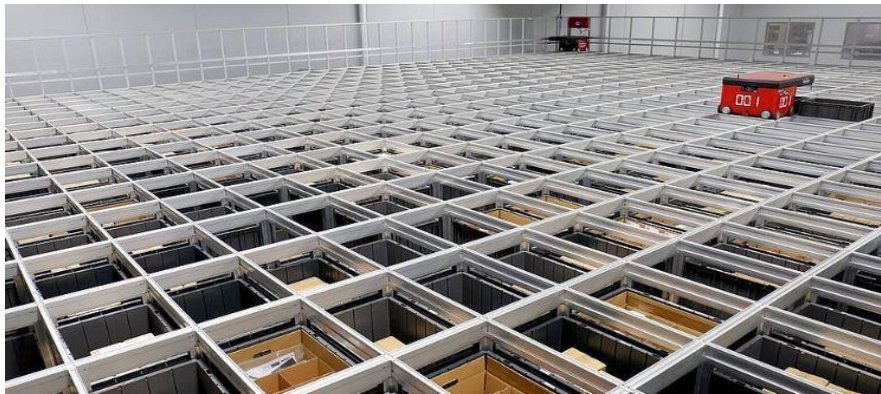
Figure 46. Structural aluminum grid.
