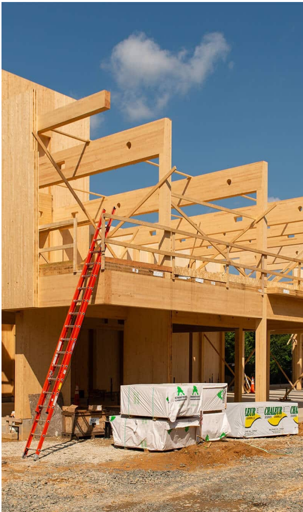
Figure 16: HITT Contracting CoLab, Glulam and CLT Structure. Reference: https://www.hitt.com/research-and-
