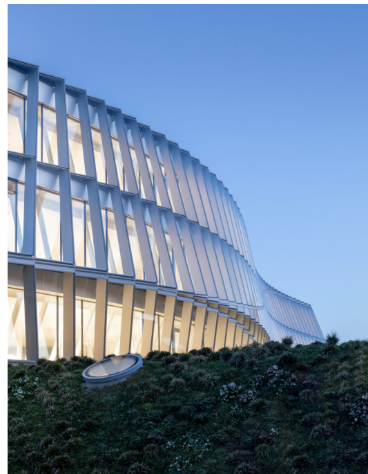
Figure 8: Glass façade showing Steel Framing. Reference: https://www.archdaily.com/919974/olympic-house-3xn
