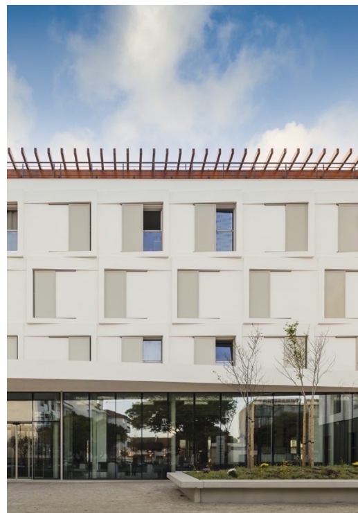
Figure 37: Front Façade. Reference: https://www.fragmentos.pt/en/projects/lombos-10
