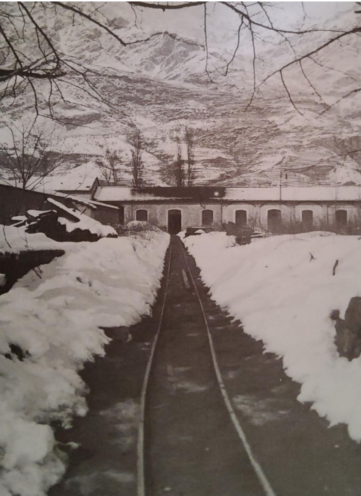
Figure 85: Siding with the Turin-Modane railway. It led to the shearing department and ended with a revolving platform. 282
