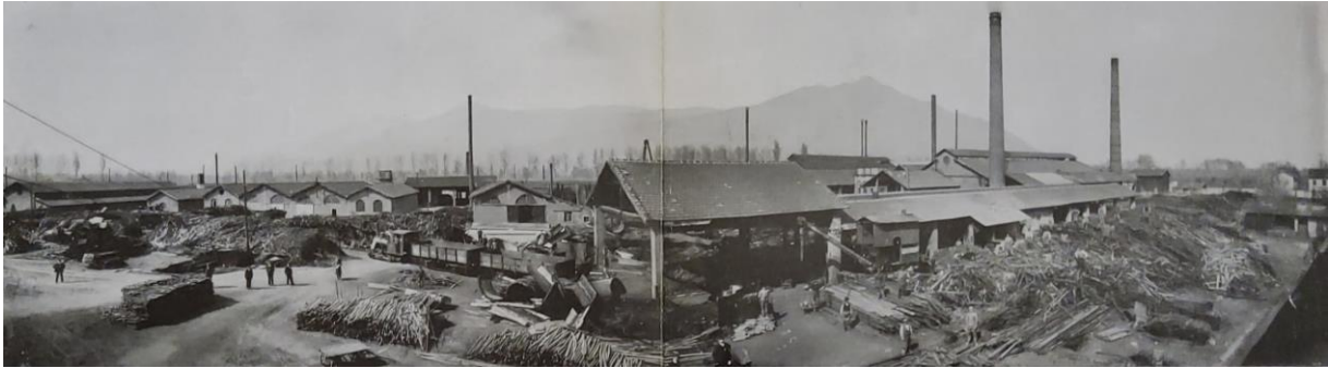
Figure 41: General view of the factory 165
