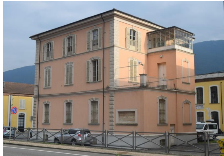
Figure 127: Current view of the office building.
