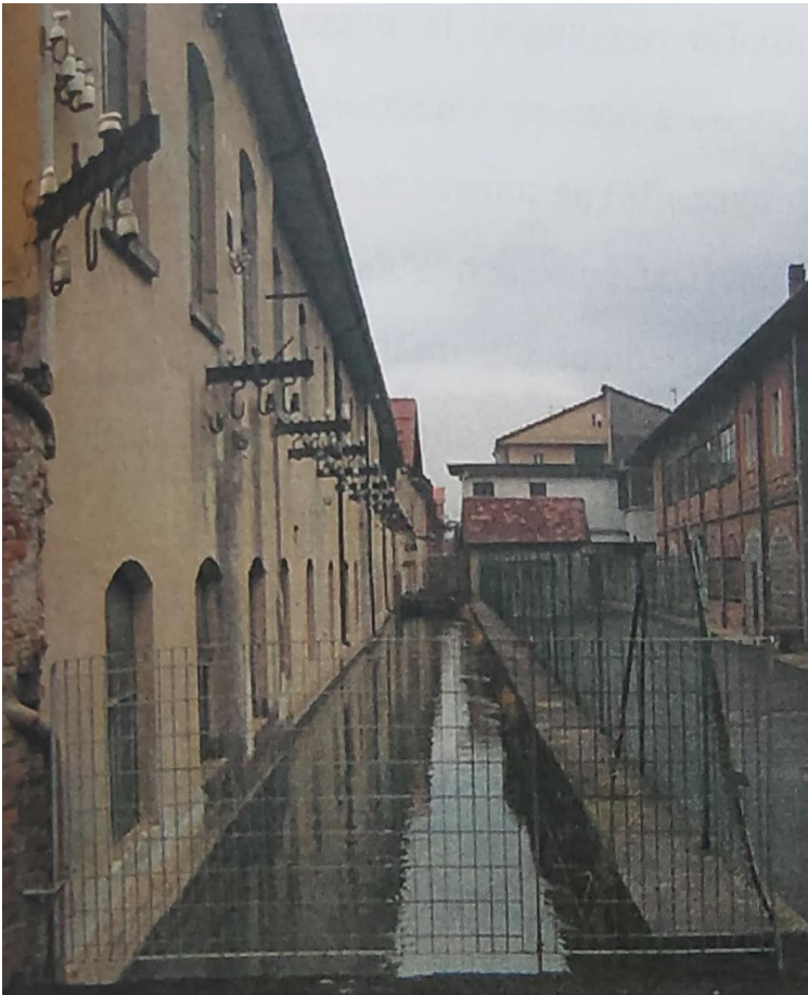
Figure 57: Southern elevation on the Cantarana bealera. 216
