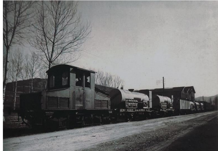
Figure 49: Internal narrow gauge track 202
