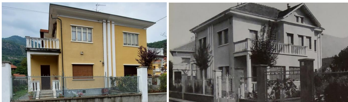
Figure 122: Current and past 316 view of the residences of Mussolini village on Via Antonio Gramsci.
