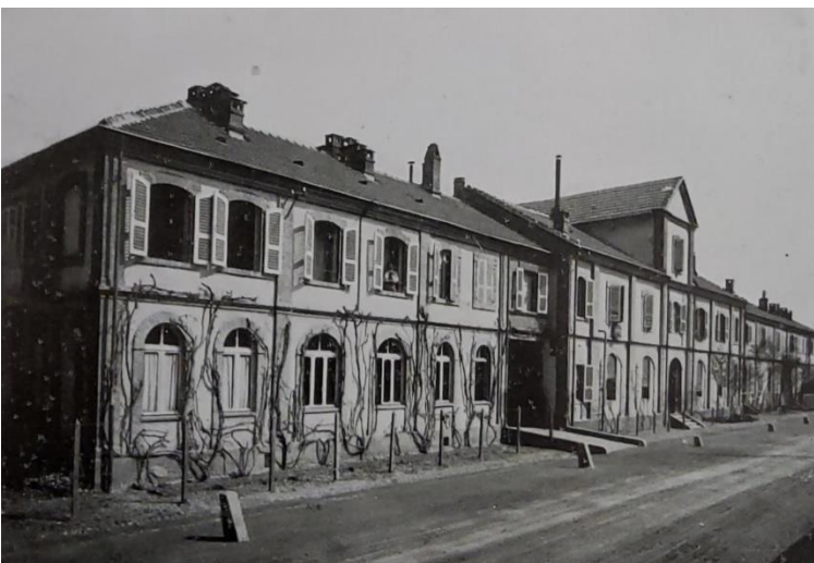
Figure 45: The former office building 191
