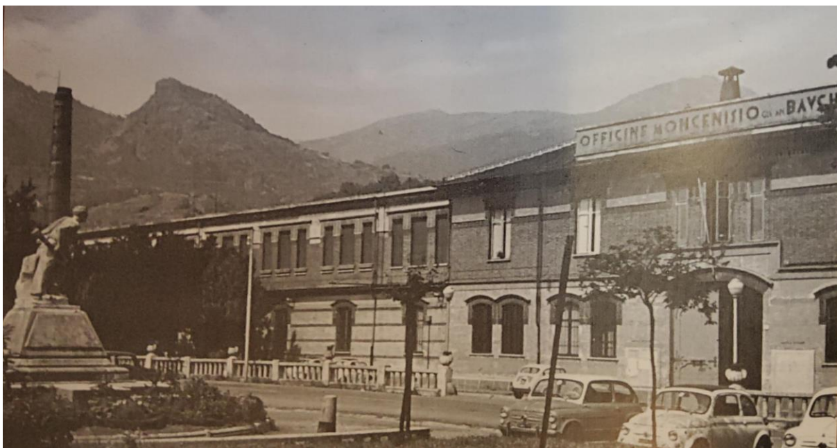
Figure 65: Main facade with the entrance and offices (post-war period). 226
