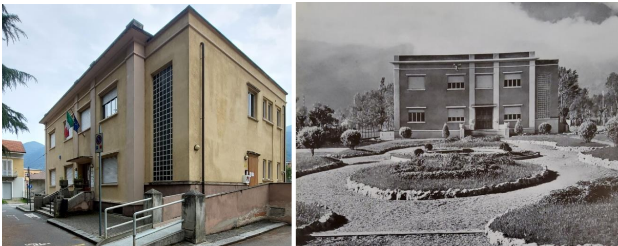
Figure 123: Current and past 317 view of the health centre.
