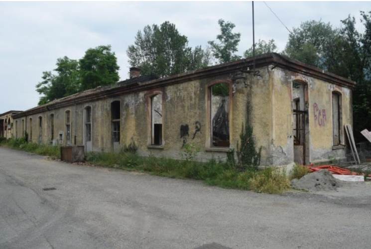
Figure 129: One of the abandoned buildings.
