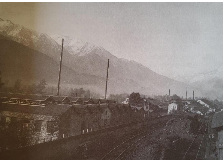
Figure 93: On the left of the photo is the tubing department; two large flywheels, placed on the external wall of the building, connected with cables to the hydraulic motor, transmitted motion to all the machines in the workshop. 291
