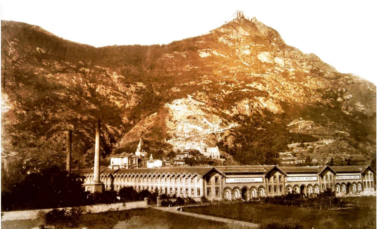
Figure 54: View of the two main fronts. 213
