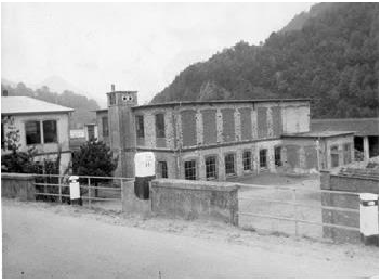
Figure 84: View of the Chianocco factory, 1955. 258
