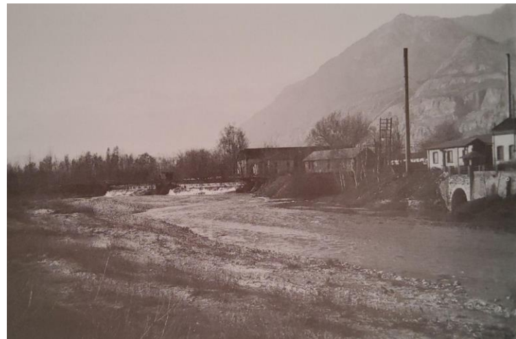
Figure 87: On the right of the photo is the unloader of the channel; above it the turbine building; to the side of this the chimney of the pickling boiler and the office building. 284
