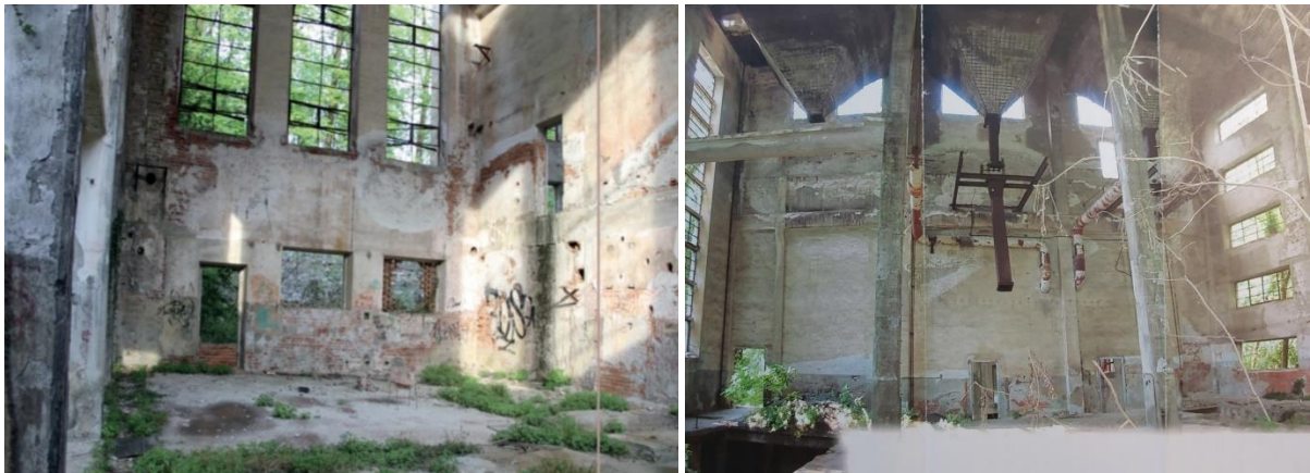
Figure 113: Current view of the thermoelectric power plant. 311
