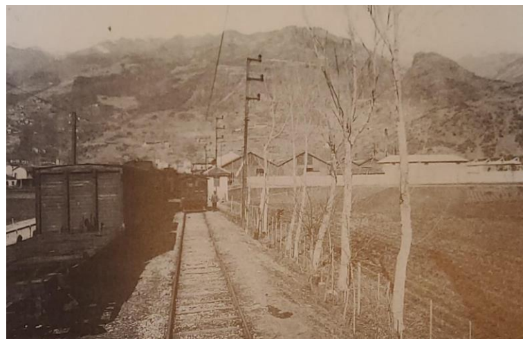
Figure 74: The connection between the plant and the Condove Chiusa di San Michele railway station. Visible, in the distance, the small engine used to transport the wagons and personnel. 239
