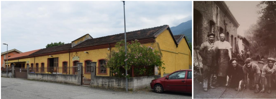
Figure 132: Current and past 319 view of the only building identified in usable condition.
