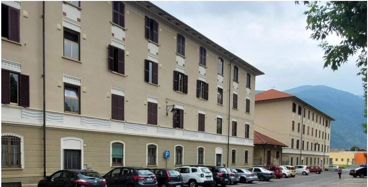
Figure 121: First constructed blocks of residences near Viale Bauchiero.
