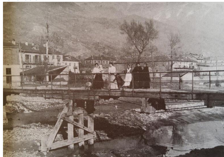
Figure 97: The bridge under construction: supported by wooden beams, later replaced with iron beams. 299
