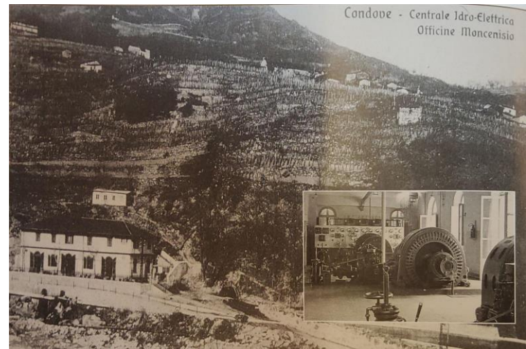
Figure 72: The hydroelectric plant on the Gravio torrent. 236
