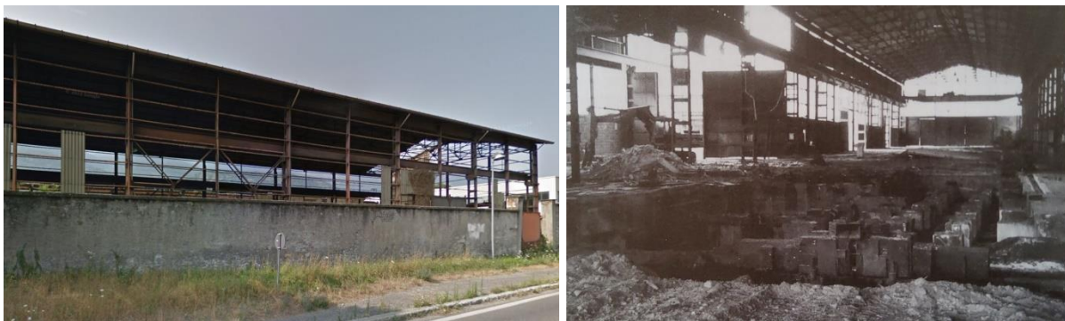
Figure 134: The rolling mill shed. 321 Currently it is almost completely demolished.
