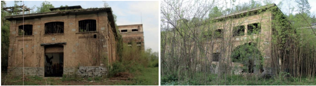
Figure 112: Current view of the factory building. 310
