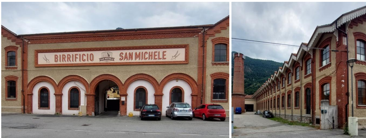
Figure 114: The facade of the factory with abundant ornaments.
