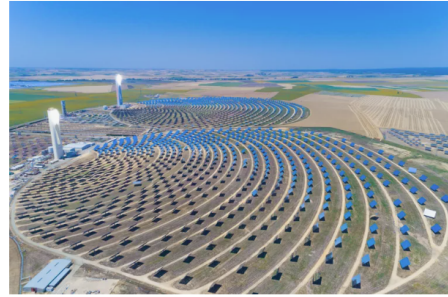
Figure 3.8: PS20 and PS10 solar tower plants, Andalusia, Spain[38]
