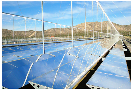
Figure 3.6: Puerto Errado 1 solar power station, Murcia, Spain[35]
