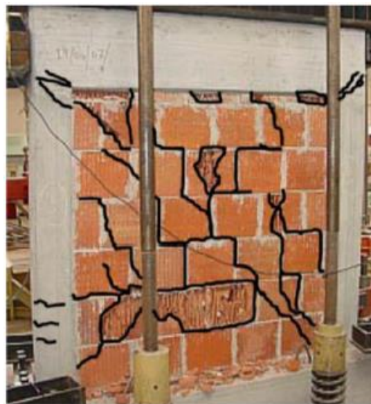
Figura 2.9 – Crack pattern a fine test del provino S1B [32]
