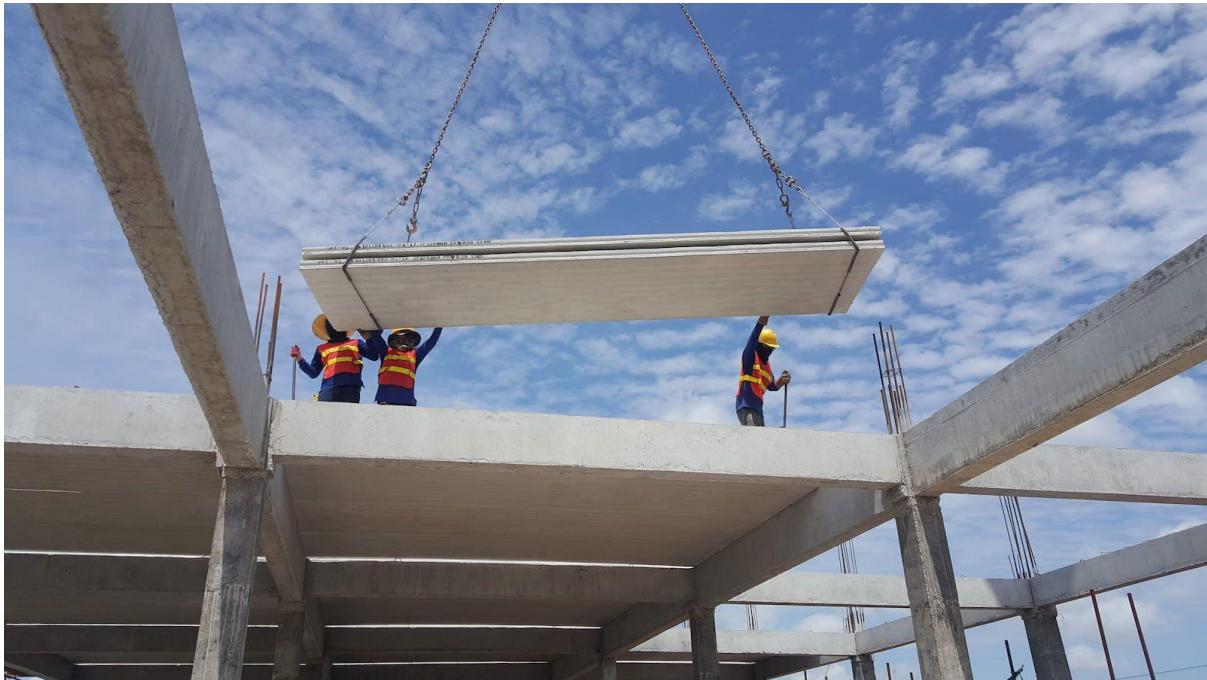
Figure 27- Installation of Precast hollow core
