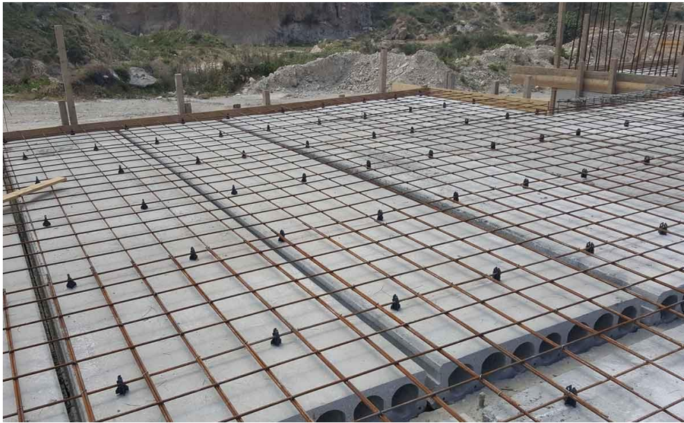
Figure 26- Precast hollow core concrete slab
