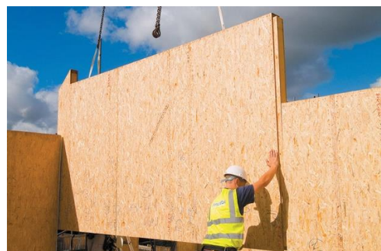
Figure 25- installing Sips panels
