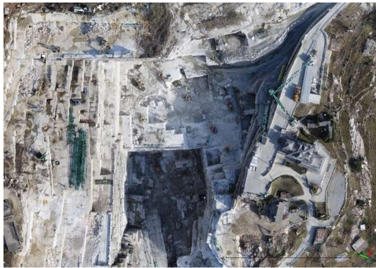
Figure 28: Analyzed excavation area.
