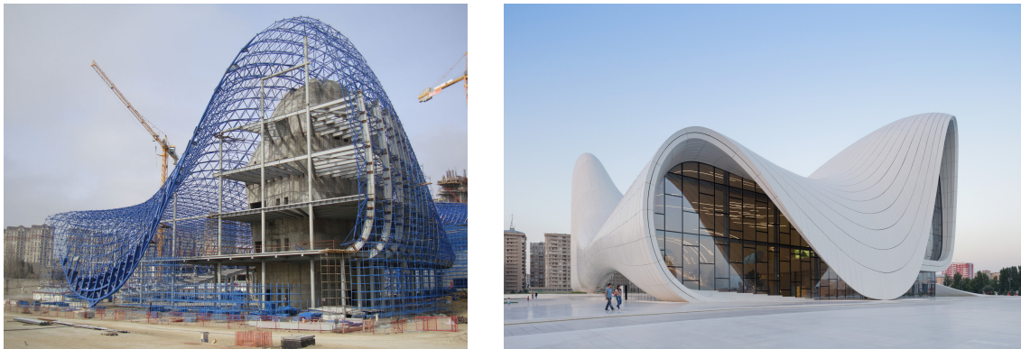
Figure 3.3: Heydar Aliyev Cultural Center underlying structural system
