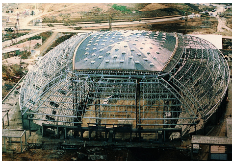
Figure 3.2: Palau Sant Jordi sporting arena structural system
