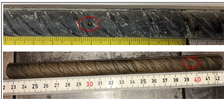
Figure 57: C4 rebar pit. Pre-cleaning (top), post-cleaning (bottom)
