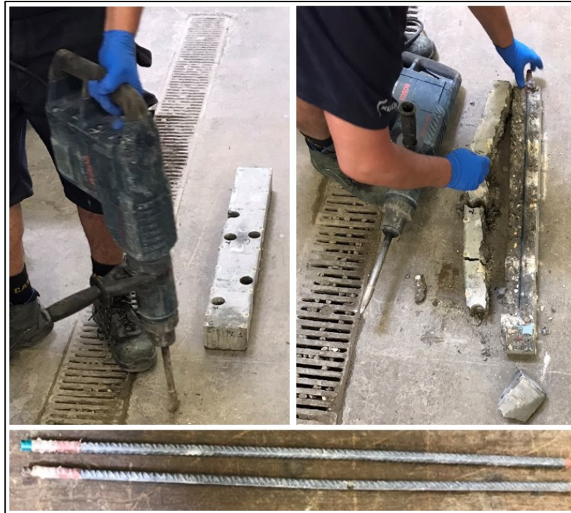
Figure 54: Samples C4 and CN3 rebar extraction
